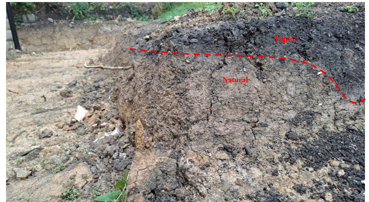
Photo 2: Cross section near building which shows nominal thickness of topsoil above natural soil.
