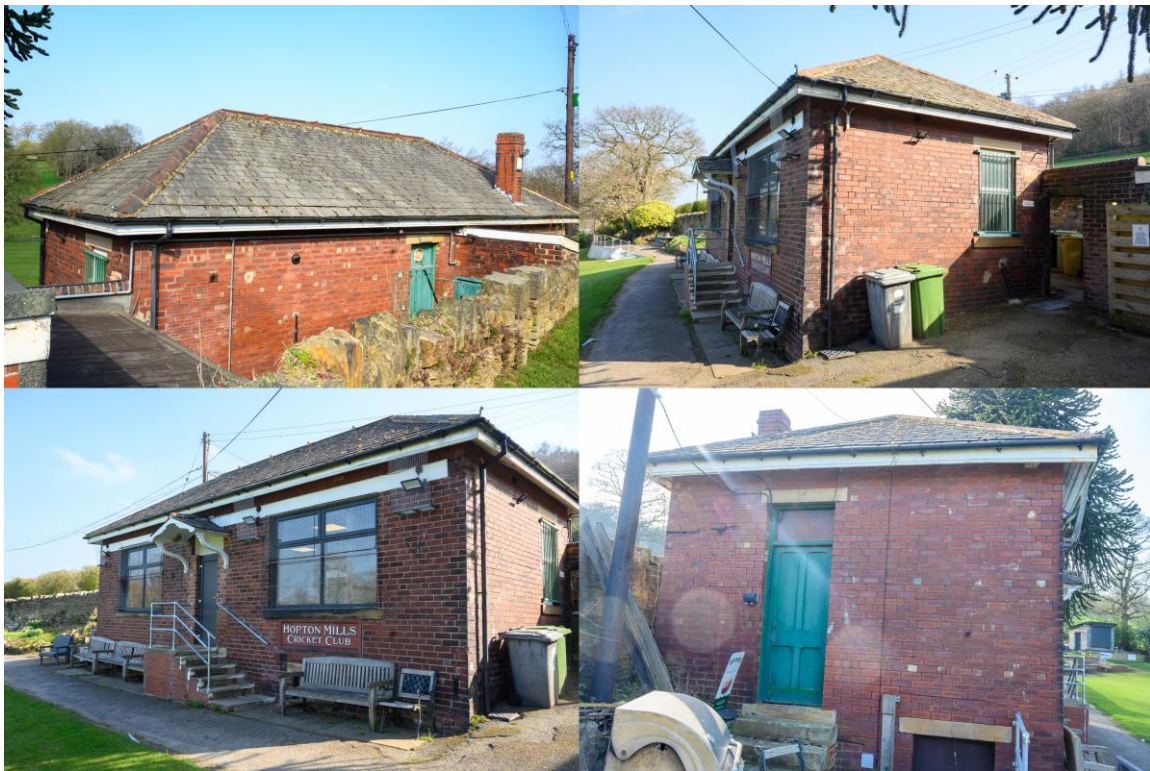
Photo 1 showing all elevations
