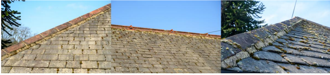
Photo 2. Showing roof and very sound ridge sections.
