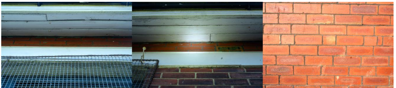
Photo 3 showing the soffits and English bond walls
