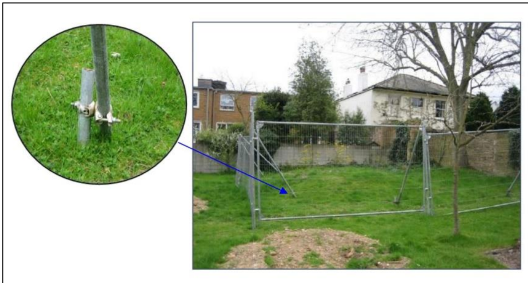
Figure A3.1: Example of mesh welded type barriers in-situ.
