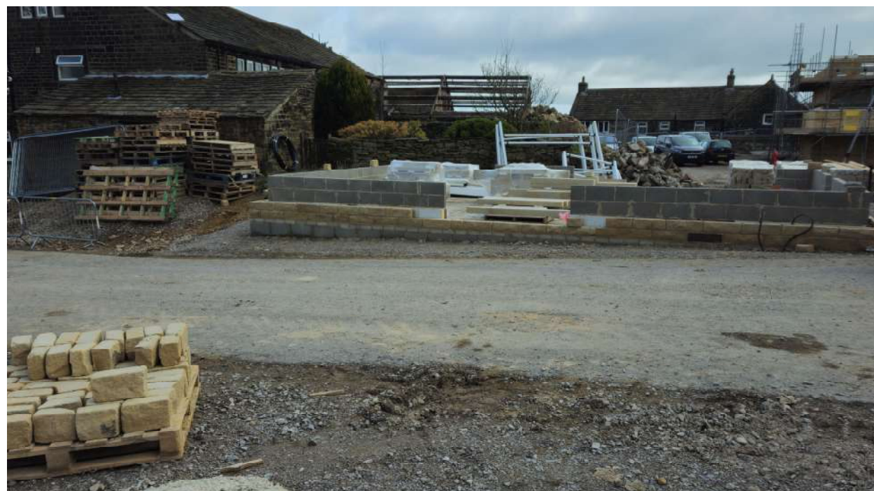
Photo 33: Large site level drop to west of site showing made ground is removed.
