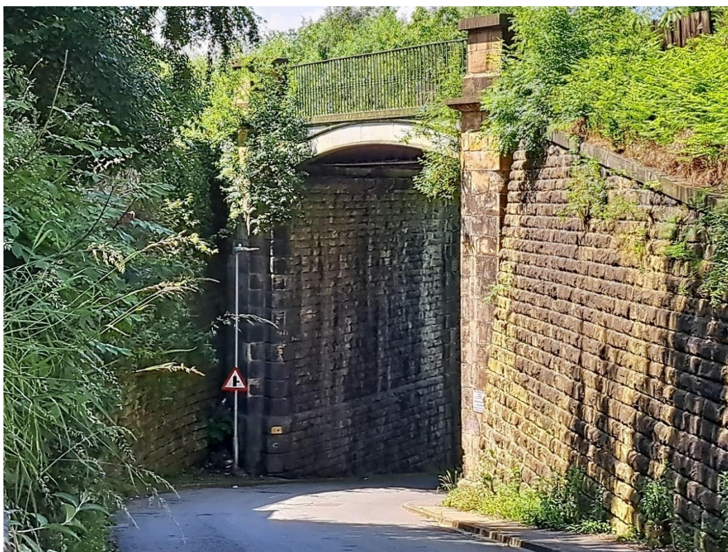
Insert 1-1 Jack Lane Underbridge (MDL1/24) – Eastern Elevation.
