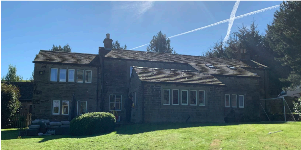
Fig 2.0 Photograph of North West Elevation
