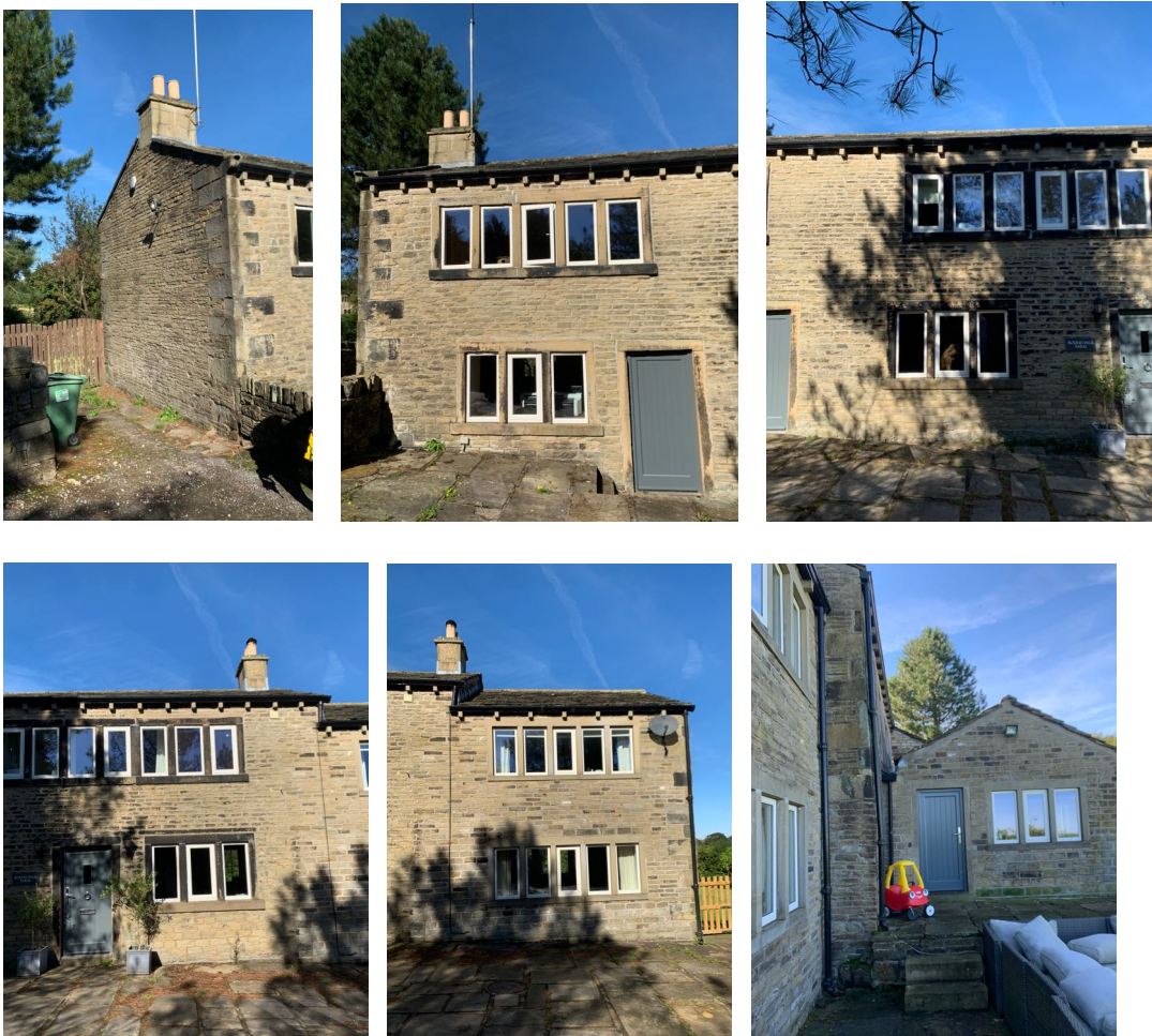
Fig 3.0 Close up Photographs of Existing Building
