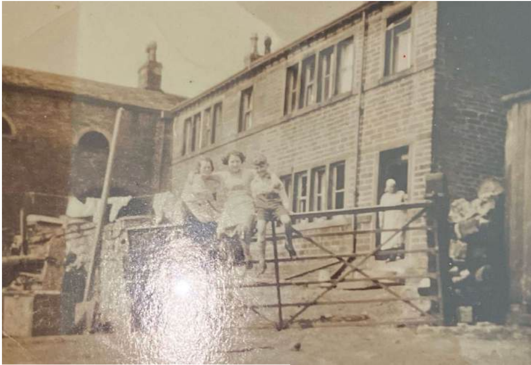
The building when it was 2 separate dwellings
