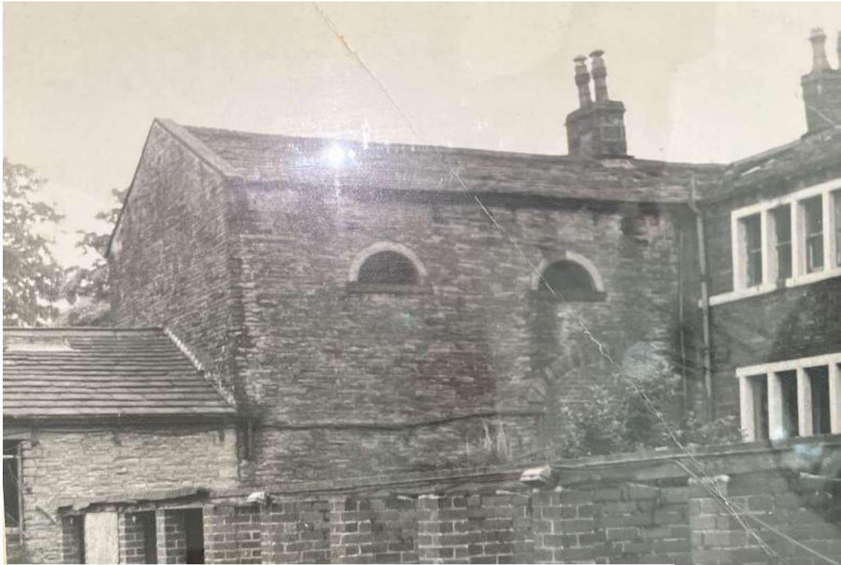
Photo of the barn which was extended and converted into a habitable area.
