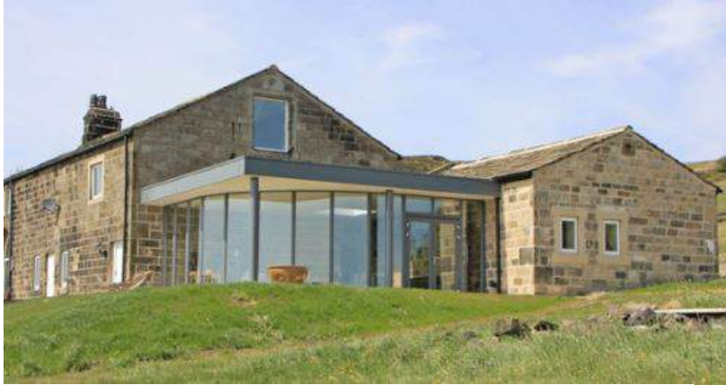
Example of contrast of heavy stone and new modern glazing
