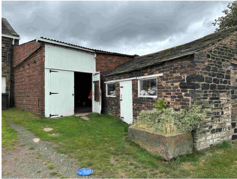
Photograph 1 – View From the South
