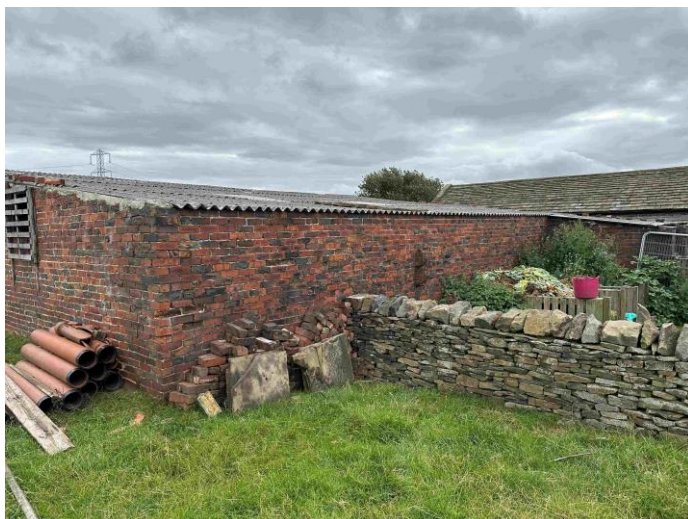
Photograph 5 – View of North West Corner
