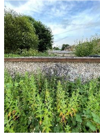
View of east wall of B4
