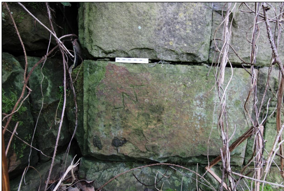
Plate 10: Example of mason's mark on southern pilaster plinth with 10cm scale (eastern elevation). View facing west (IMG_1709)
