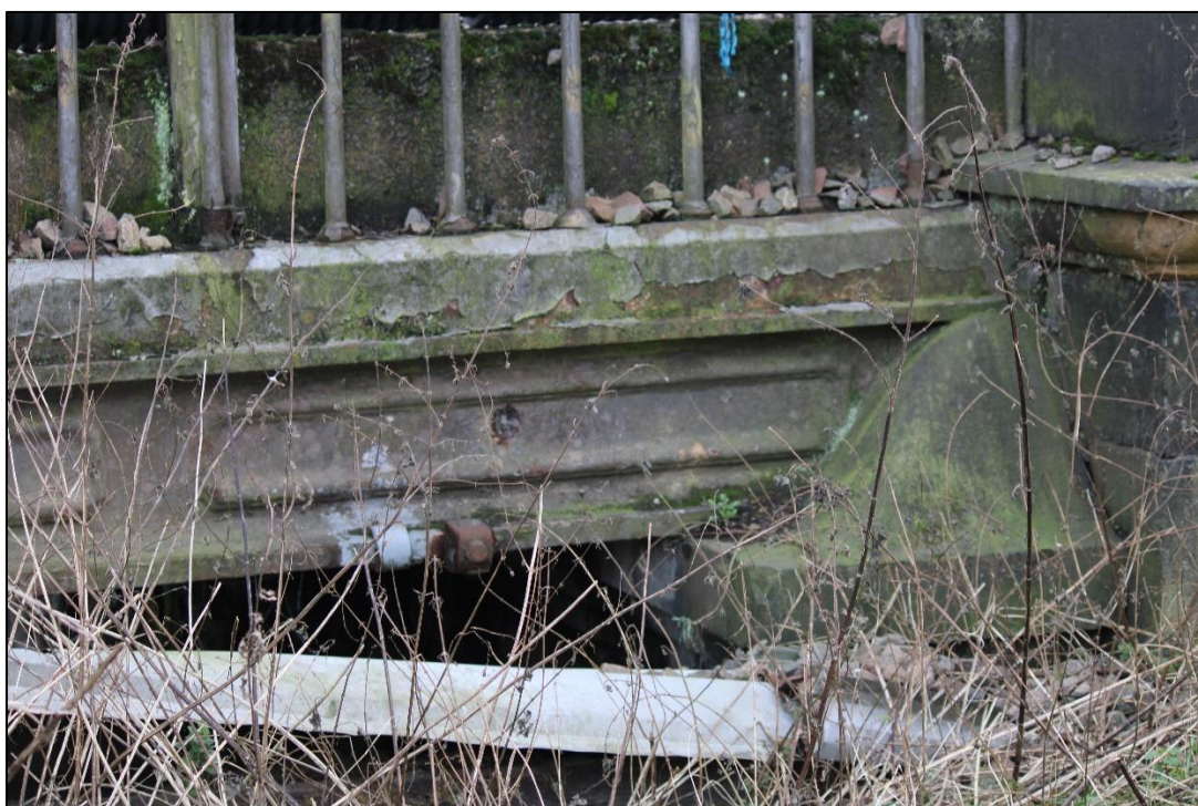
Plate 44: Southern end of embellished fascia beam with robust moulded ashlar cornice (right) (western elevation). View facing south-east (IMG_1784)
