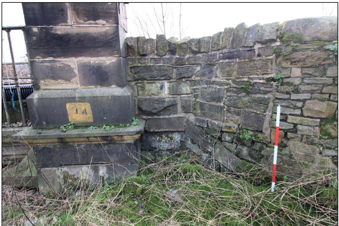
Plate 40: Southern wing wall with later boundary wall addition with 1m scale (western elevation). View facing east (IMG_1790)
