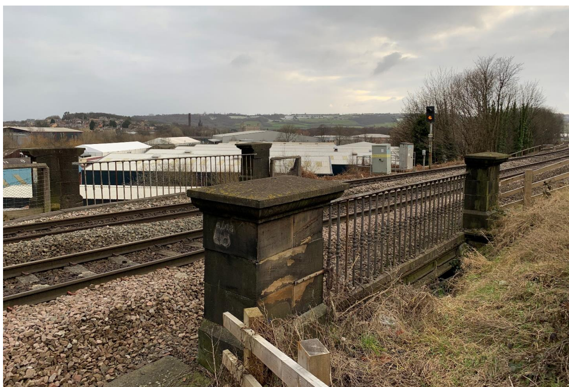
Insert 4-5 Toad Holes Underbridge (MDL1/12) - infilled north western approach from Watergate Road.
