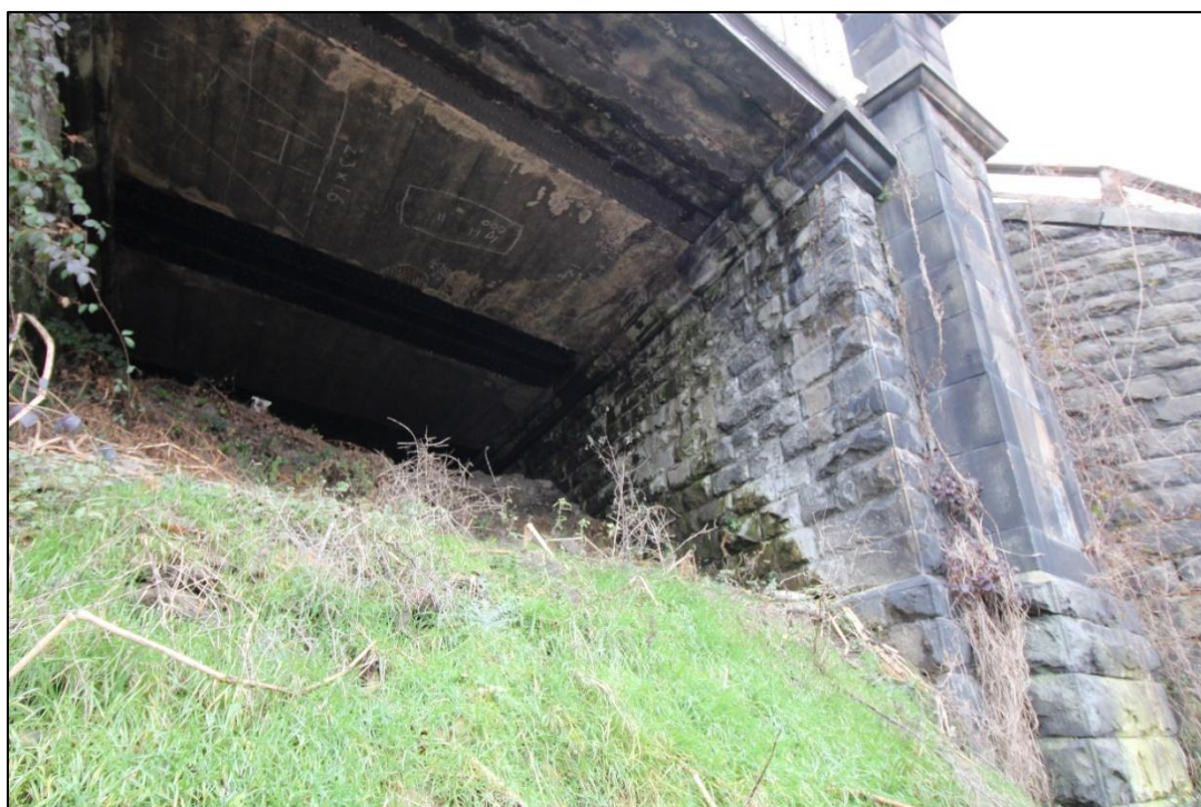
Plate 23: Internal elevation of northern abutment. View facing north-west (IMG_1684)
