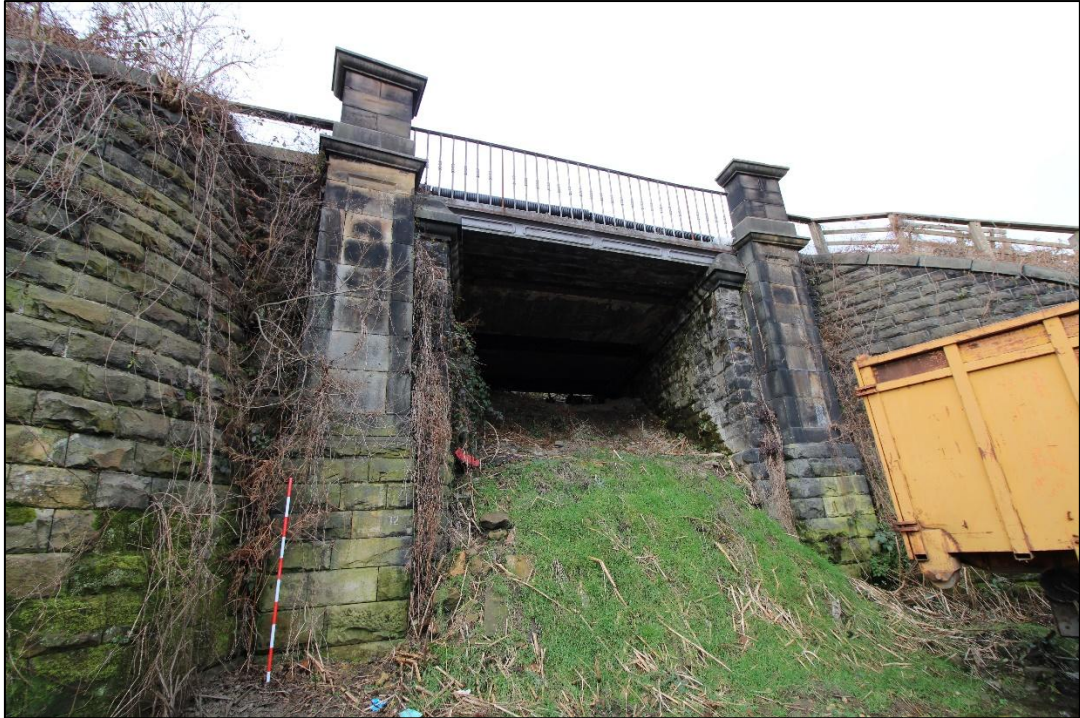
Plate 8: Eastern elevation of Toad Holes Underbridge (MDL1/12) with 2m scale. View facing north-west (IMG_1811)
