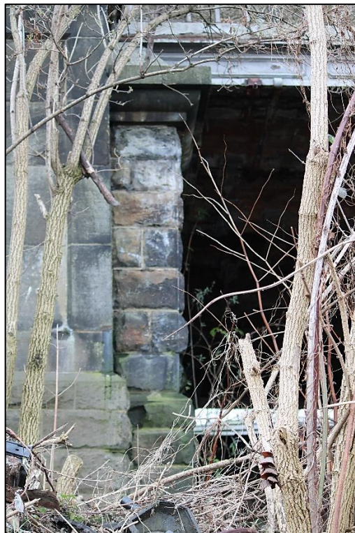
Plate 31: Southern abutment (eastern elevation). View facing north-west
