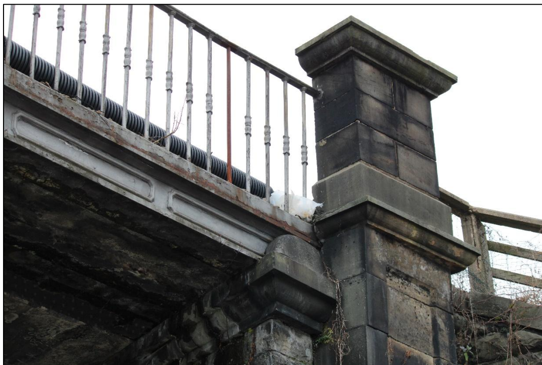
Plate 12: Northern parapet end pillar (eastern elevation). View facing north (IMG_1689)
