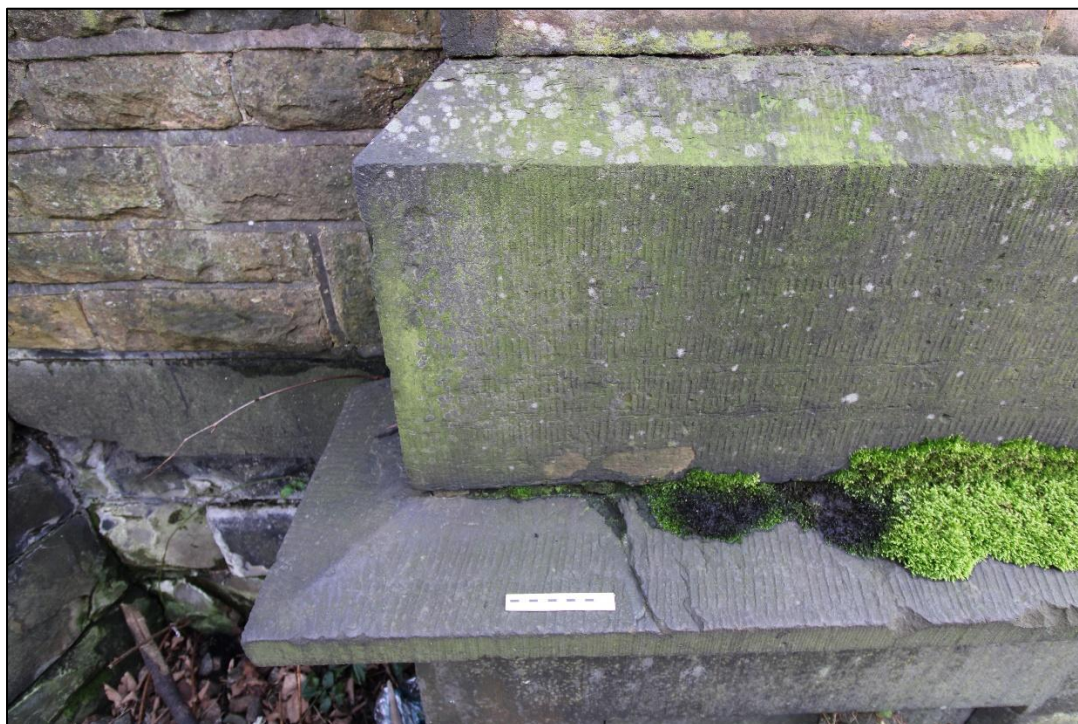
Plate 41: Vertical tooling marks on pilaster cornice and parapet end plinth with 10cm scale (western elevation). View facing south-east (IMG_1775)
