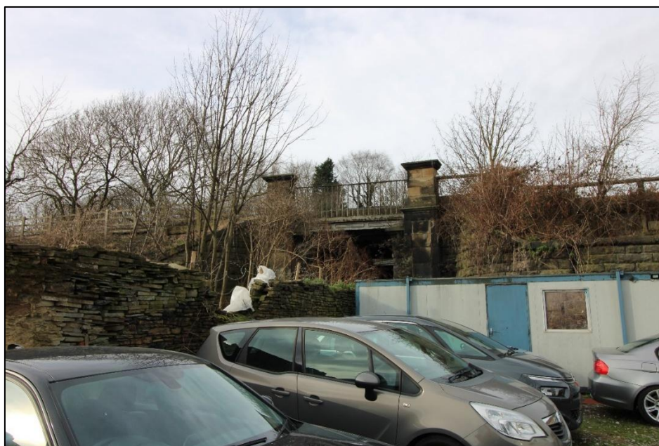
Plate 28: Eastern elevation of Ming Hill Underbridge (MDL1/14). View facing west
