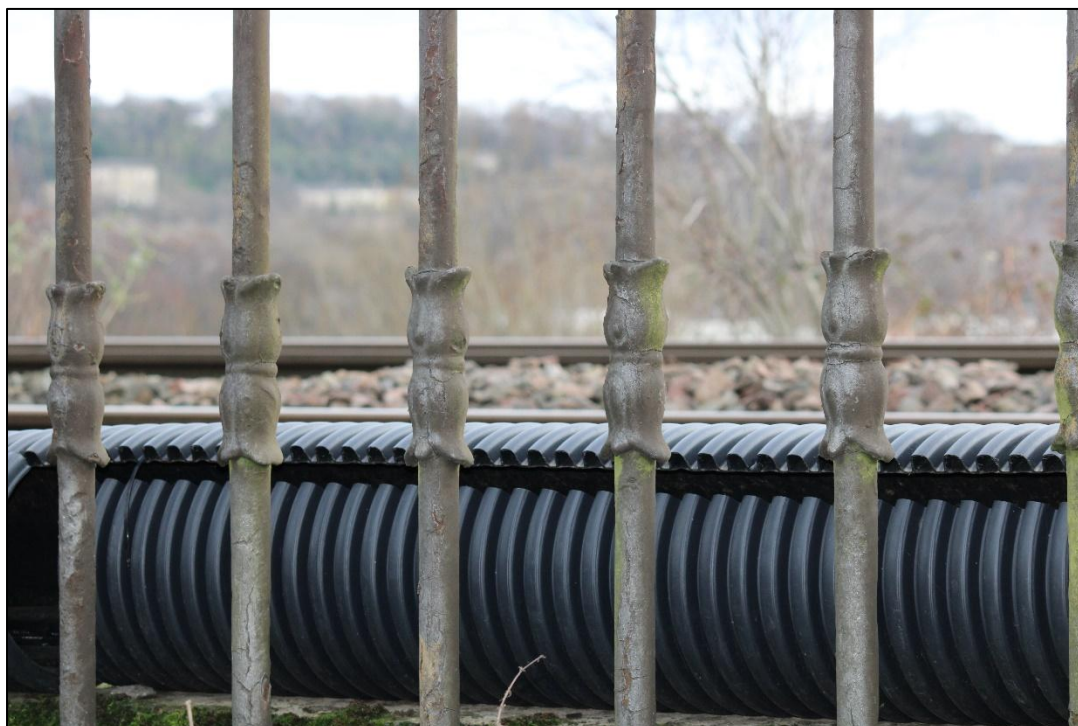
Plate 42: Tulip-formed mid-sections of balusters (western elevation). View facing east (IMG_1793)
