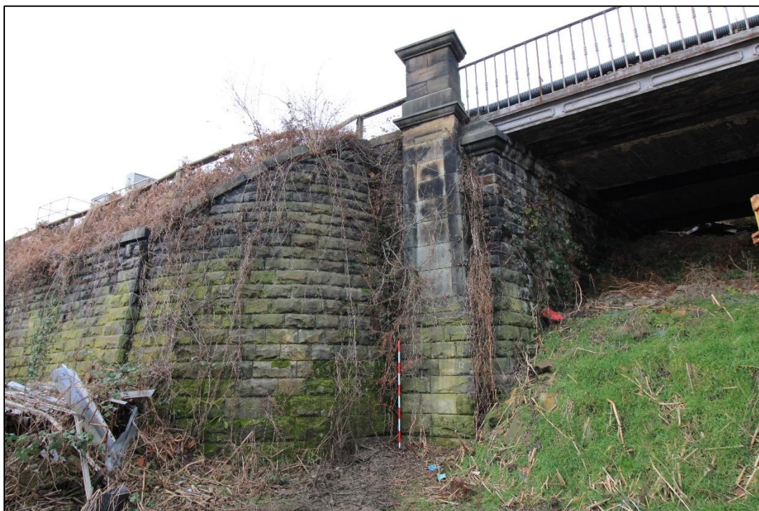
Plate 17: Southern wing wall with 2m scale (eastern elevation). View facing south-west (IMG_1809)
