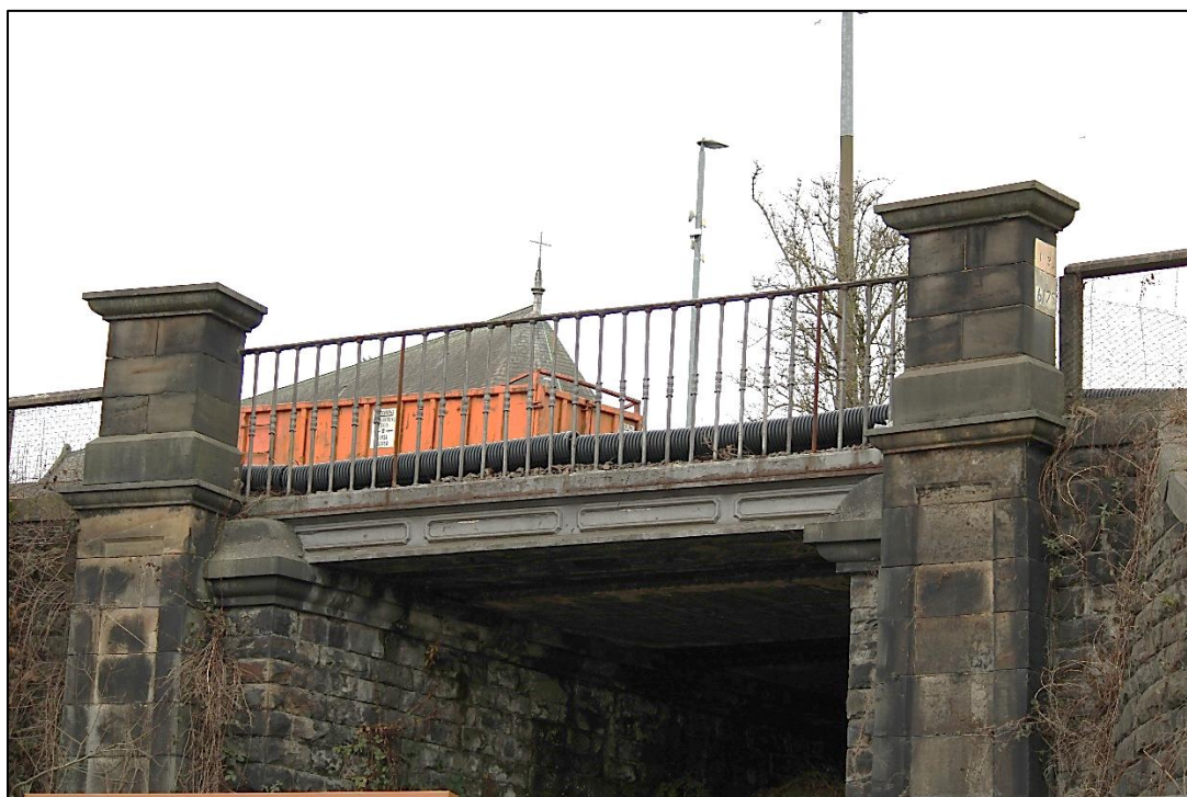
Plate 15: Cast iron level beam bridge deck (eastern elevation). View facing south-west (IMG_1664)
