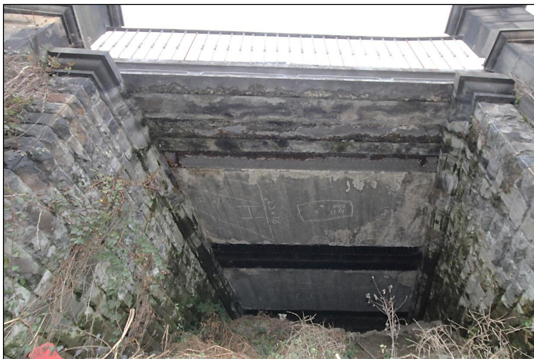
Plate 26: Underside of bridge deck with original cast-iron edge beam (top) and twentieth century alteration (centre) (IMG_1685)
