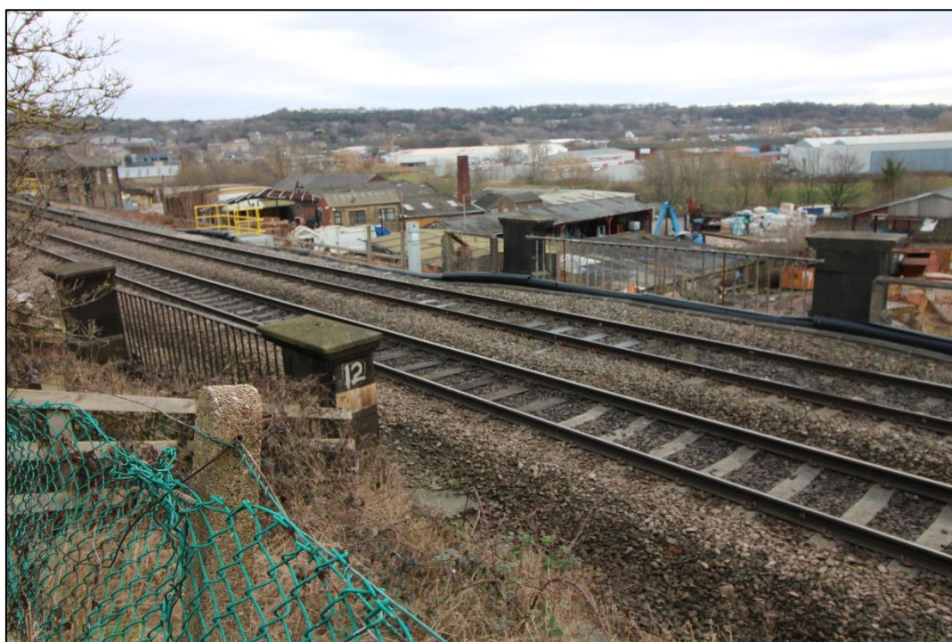
Plate 21: Western elevation of Toad Holes Underbridge (MDL1/12) (left) and rear of eastern elevation (right). View facing north-east (IMG_1657)
