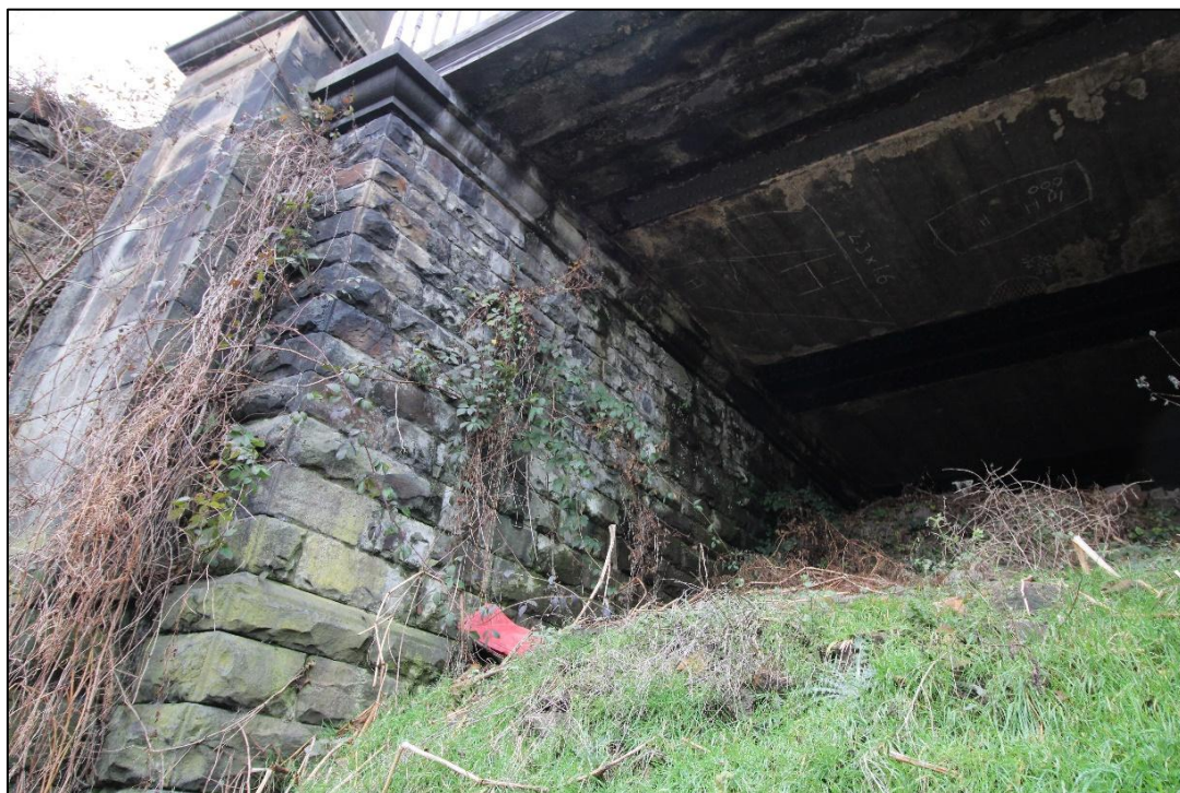
Plate 22: Internal elevation of southern abutment. View facing south-west (IMG_1682)
