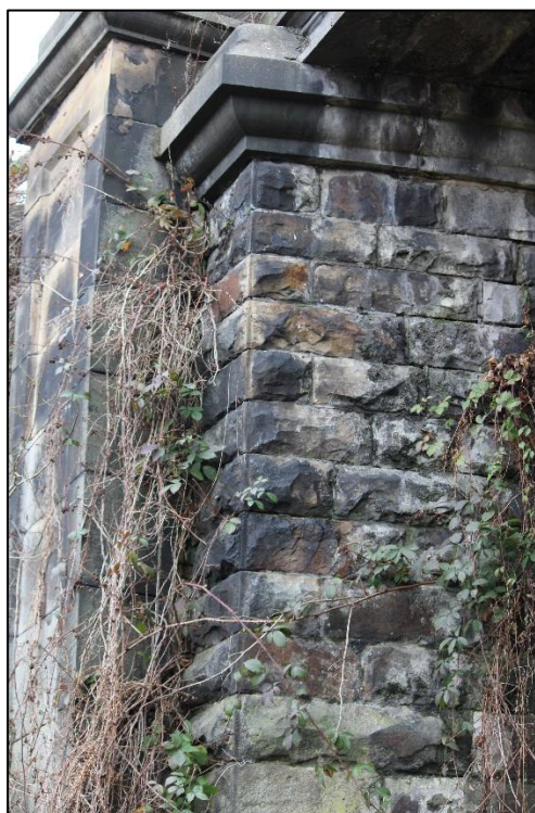
Plate 13: Southern abutment. View facing south-west (IMG_1698)
