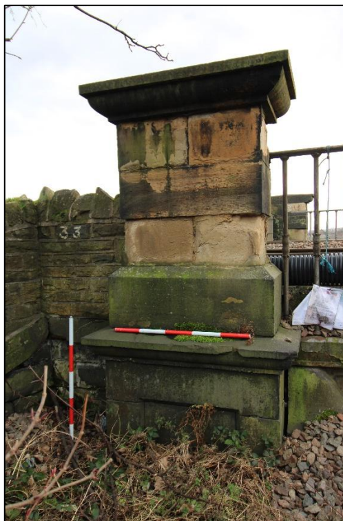
Plate 37: Northern pilaster and parapet end pillar with 2 x 1m scales (western elevation). View facing east (IMG_1773)
