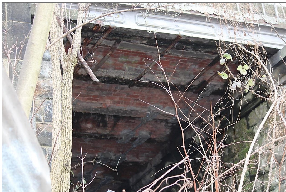
Plate 45: Brick jack arches and riveted steel girders beneath deck. View facing north-west (IMG_1745)
