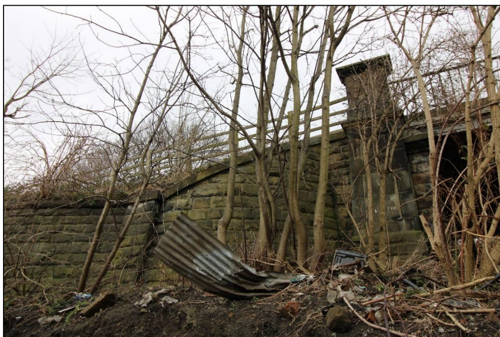
Plate 35: Southern wing wall with shallow buttress (eastern elevation). View facing west (IMG_1750)
