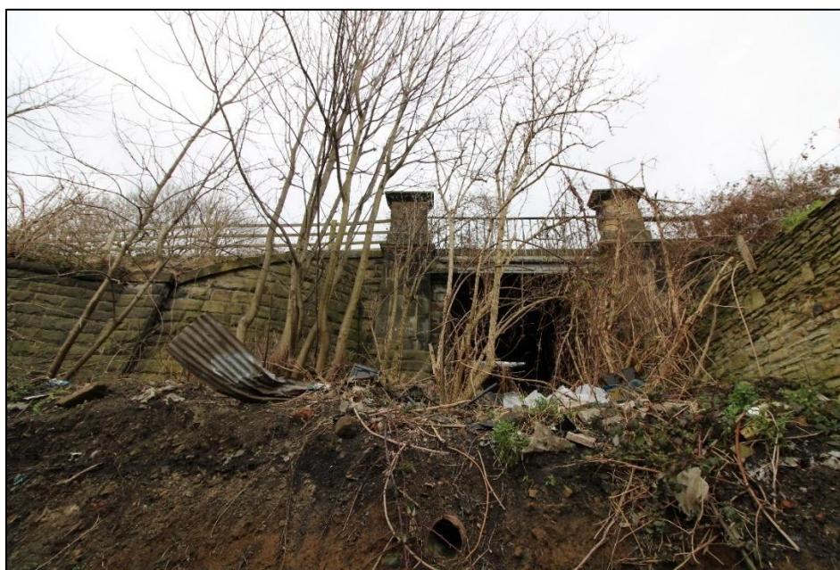
Plate 27: Eastern elevation of Ming Hill Underbridge (MDL1/14). View facing north-west
