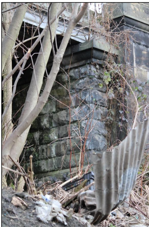
Plate 32: Northern abutment (eastern elevation). View facing north
