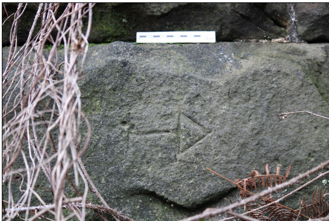
Plate 19: Example of mason's mark on southern wing wall with 10cm scale (eastern elevation). View facing south-west (IMG_1693)
