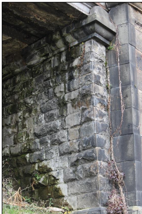
Plate 14: Northern abutment. View facing north-west (IMG_1696)
