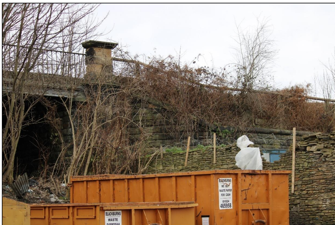
Plate 33: Attached rubble sandstone wall aligned north-west / south-east (lower centre / right). View facing north
