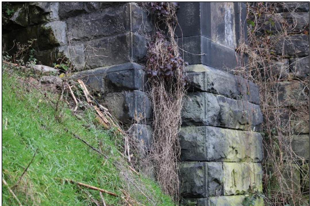
Plate 9: Example of tooled margins on northern pilaster plinth and plinth of northern abutment (eastern elevation). View facing north (IMG_1695)
