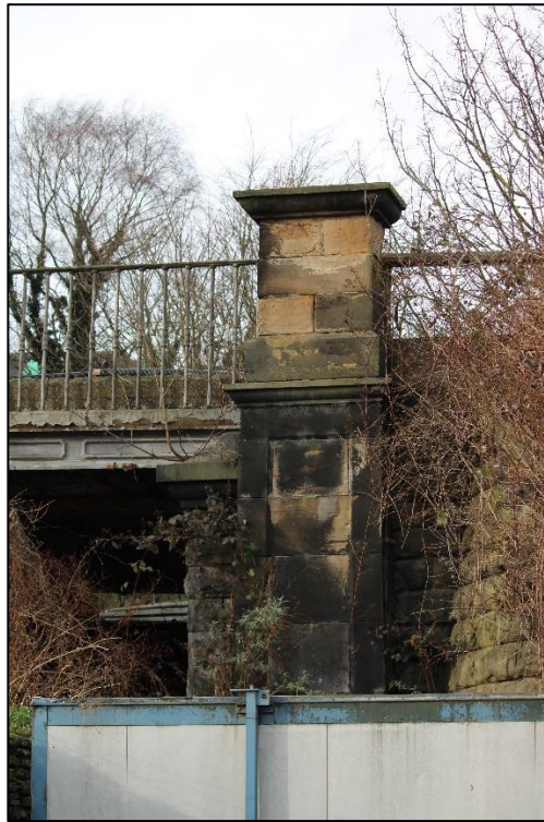
Plate 30: Northern pilaster (eastern elevation). View facing north-west
