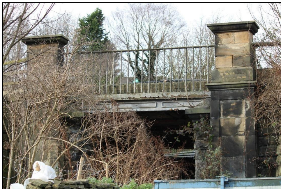
Plate 34: Cast-iron level beam bridge deck (eastern elevation). View facing west
