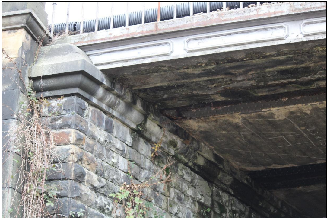
Plate 24: Moulded ashlar cornice above southern abutment. View facing south-west (IMG_1692)
