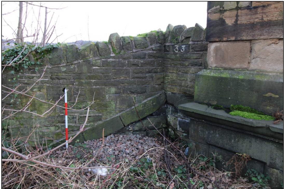
Plate 39: Northern wing wall with later boundary wall addition with 1m scale (western elevation). View facing north-east (IMG_1772)
