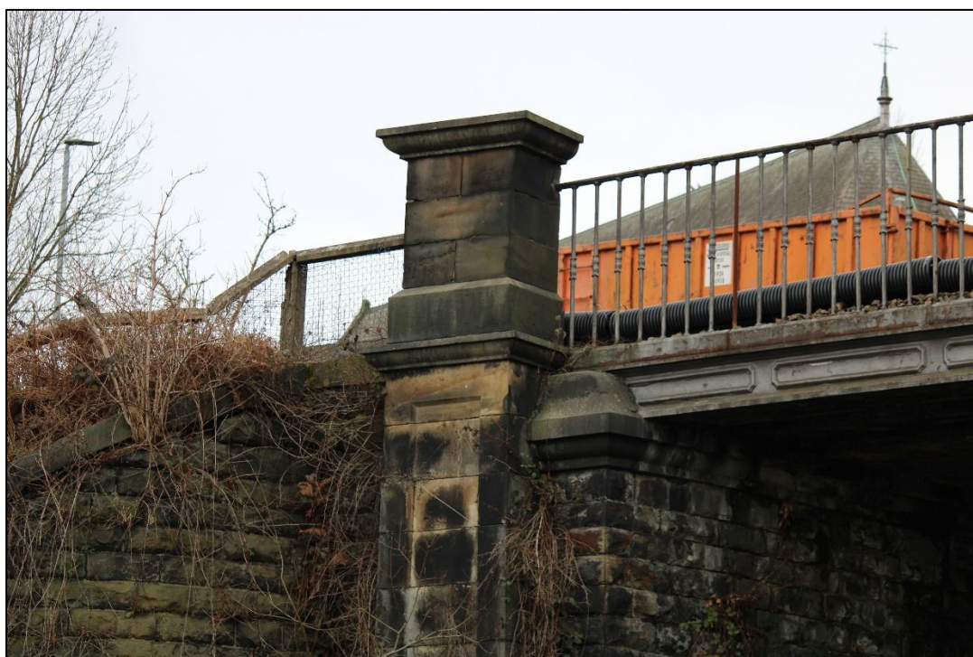
Plate 11: Southern parapet end pillar (eastern elevation). View facing south-west (IMG1663)
