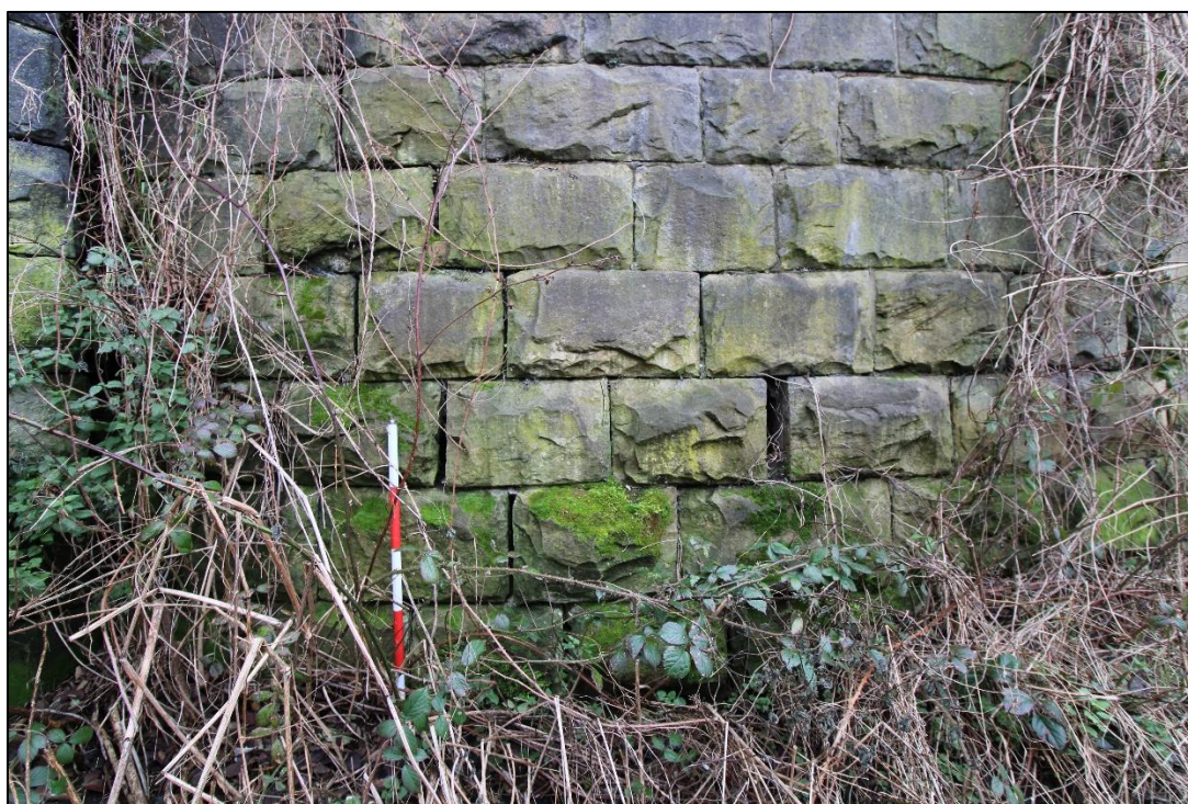
Plate 20: Stones at base of northern abutment with 1m scale (eastern elevation). View facing north-east (IMG_1710)
