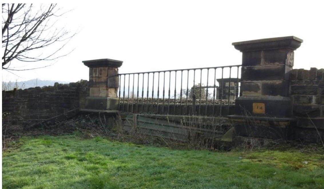
Insert 4-7 Ming Hill Underbridge (MDL1/14) – north-western infilled side of structure.
