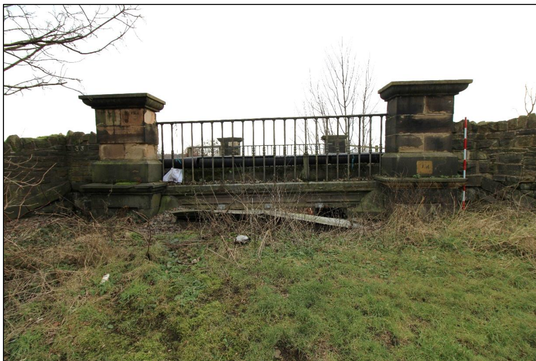
Plate 36: Western elevation of Ming Hill Underbridge (MDL1/14) with 2m scale. View facing south-east (IMG_1764)
