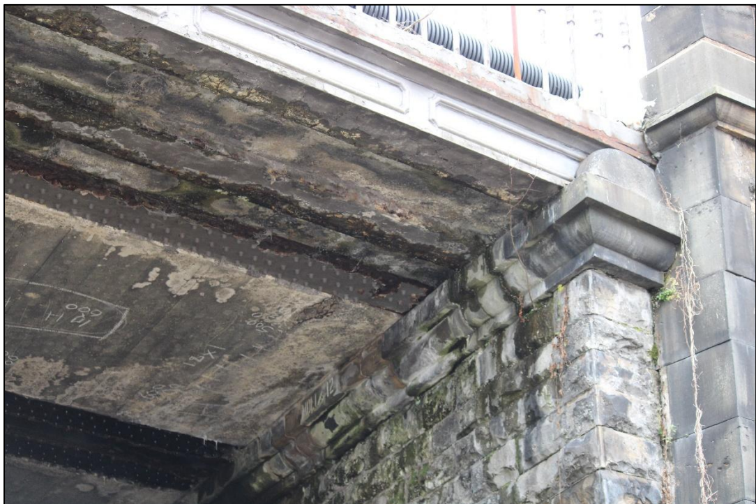
Plate 25: Moulded ashlar cornice above northern abutment. View facing north-west (IMG_1690)
