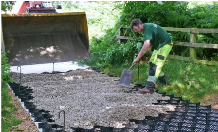
Figure 2. Example Cellular Confinement System (CCS)
