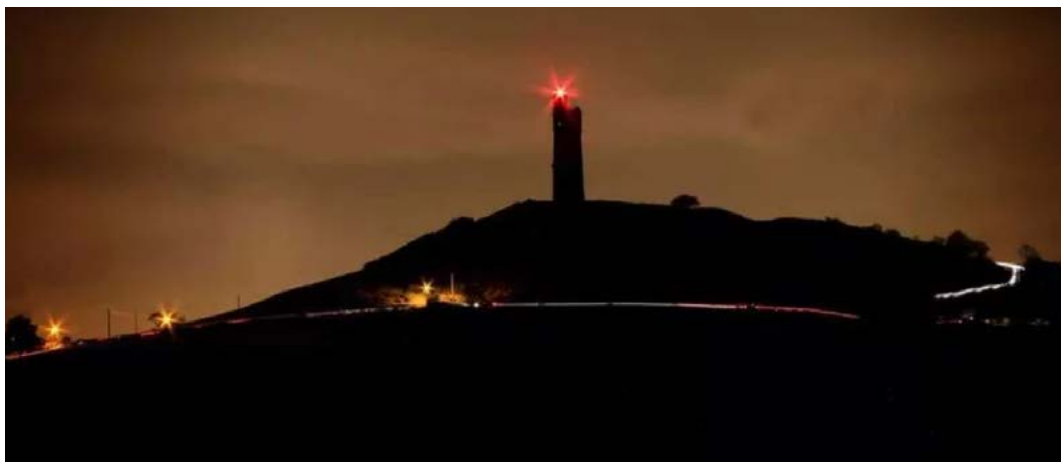
fig.5.16 Night view of Castle Hill as existing
