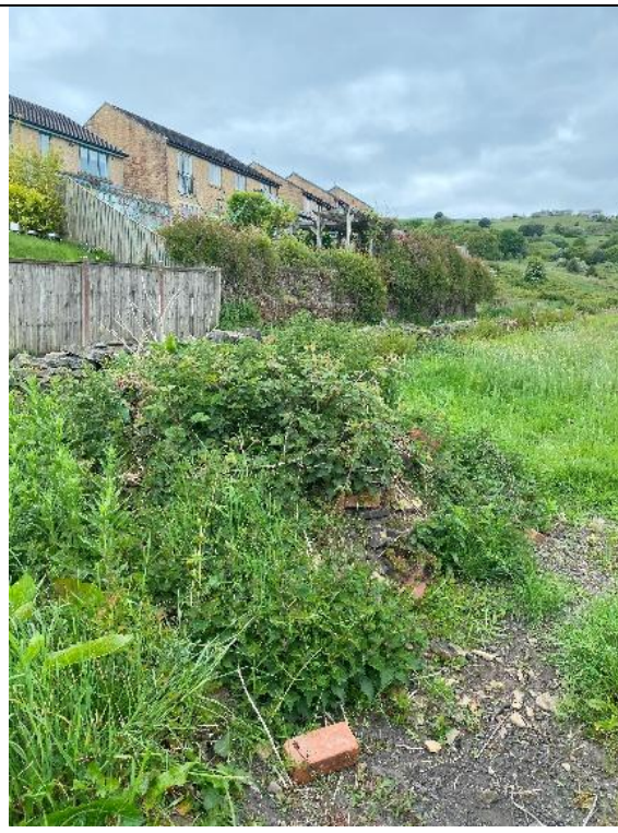
Photograph 2 – Rubble Pile (TN1)
