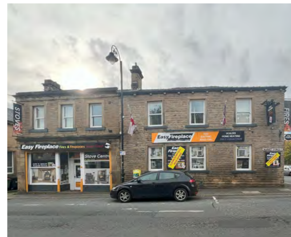
Photograph of existing North facing elevation.
