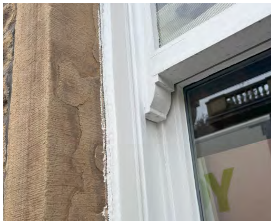
Photograph showing existing Sash Window - detailing to remain.
