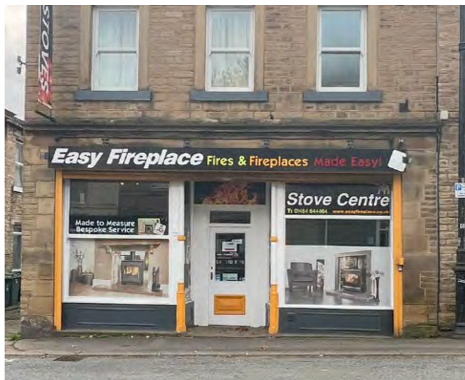
Photograph of site entrance from Market Street
