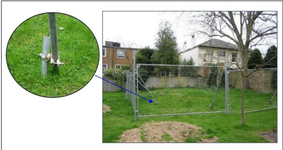
Figure A3.1: Example of mesh welded type barriers in-situ.
