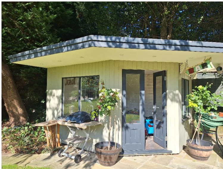
Figure 9 General view of building 1
