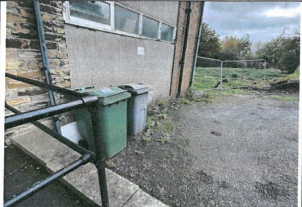
Chainage 13.2 – End of ramp. Start of unsealed surface on left hand side
