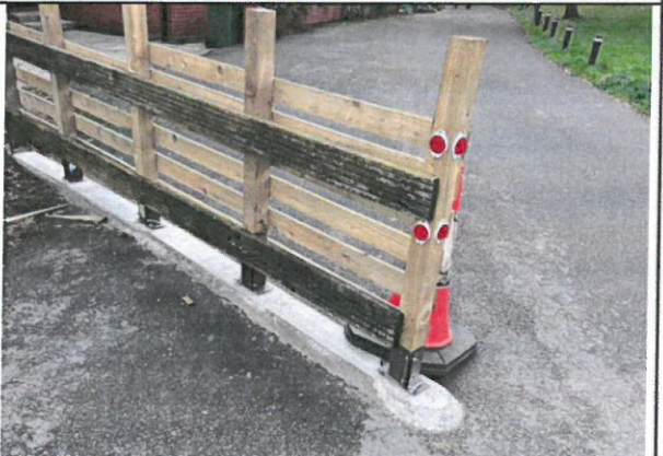
Chainage 33.6 – Start of post and rail fence on left hand side – no obvious defects
