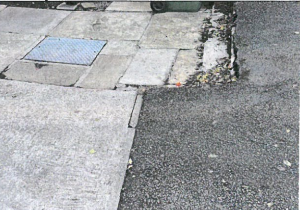
Chainage 37.6 to 42.8 – No defects in driveway
