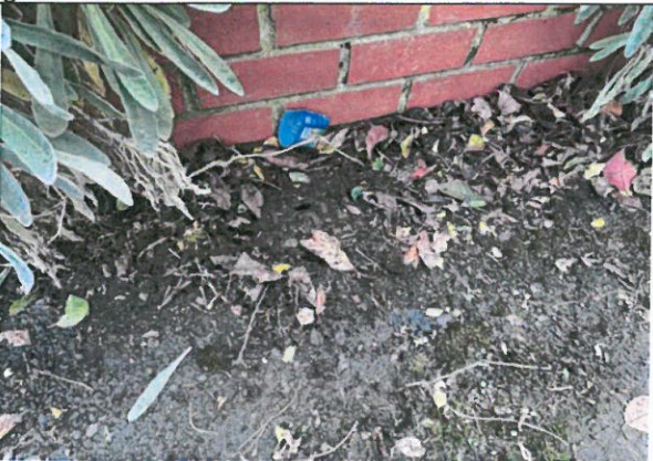
Chainage 49.6 – Small inspection chamber adjacent to boundary wall
