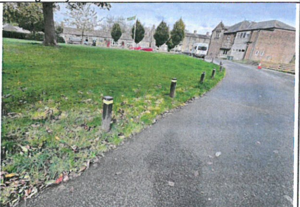
Chainage 3 to 55 – 20no bollards in verge adjacent to access road. All in good condition and structurally sound
