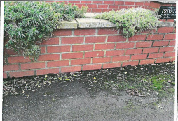
Chainage 44.5 to 55 – Property boundary wall – good condition
