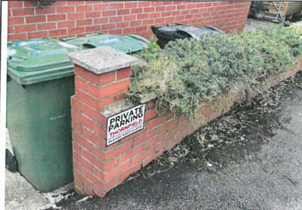
Chainage 44.5 to 55 – Property boundary wall – good condition
