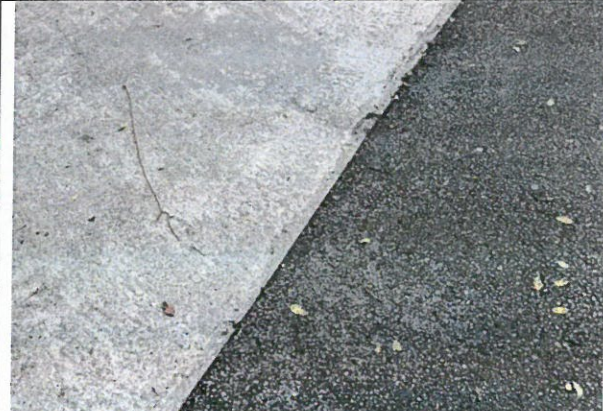
Chainage 37.6 to 42.8 – No defects in driveway
