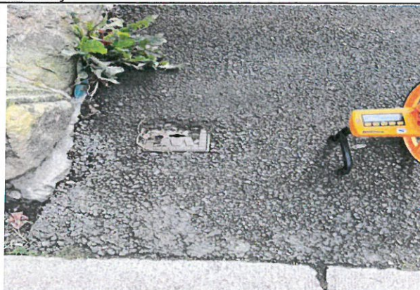
Chainage 0.5 – Water stop valve to left hand side – good condition
