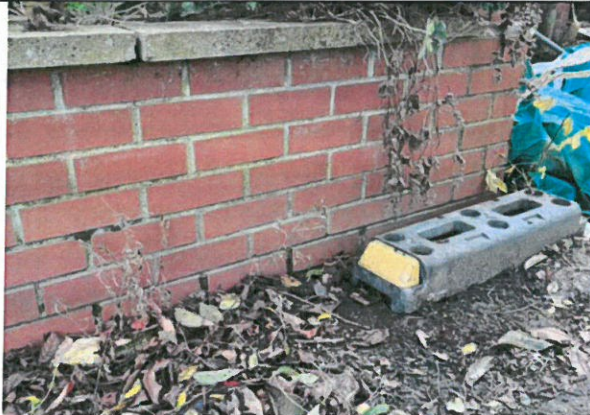
Chainage 44.5 to 55 – Property boundary wall – good condition
