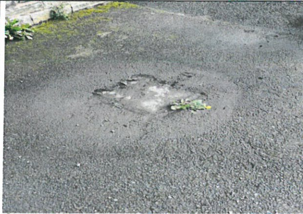
Chainage 5.3 – Inspection chamber to left hand side – good condition
