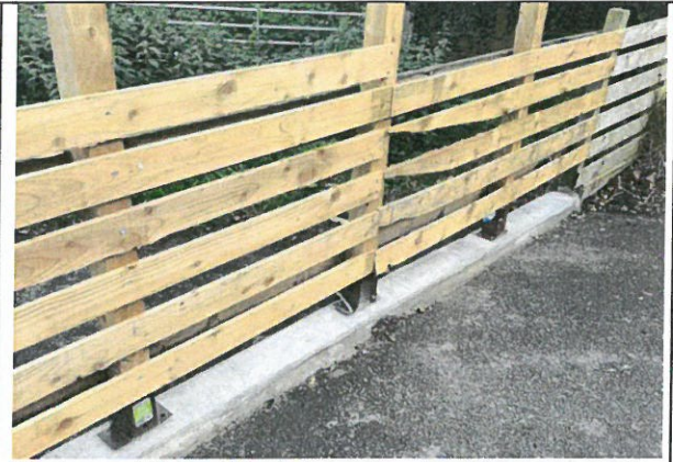
Chainage 33.6 – Start of post and rail fence on left hand side – no obvious defects
