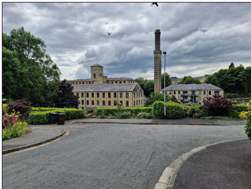
Plate 15: View looking south-west from the end of Lea Side Gardens showing part of the Parkwood Mills complex including the landmark chimney
