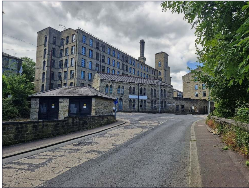
Plate 10: View looking north-west showing some of the buildings at Parkwood Mills, with the proposed development site to left of photograph
