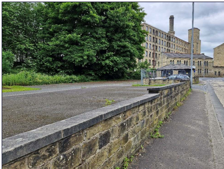
Plate 5: View looking north-west along the boundary wall on Grove Street towards Parkwood Mills
