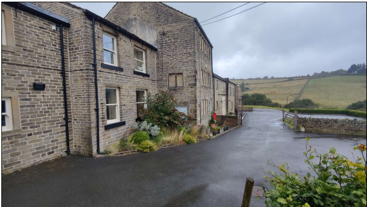
View of New Close Farm Cottage from the north elevation of the building subject to this application
