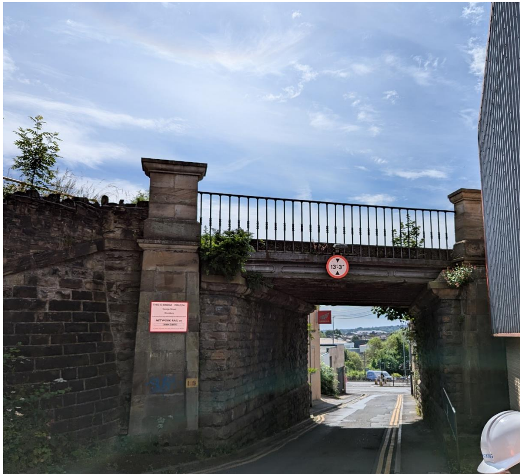
Insert 4-4 George Street Underbridge (MDL1/16), north elevation
