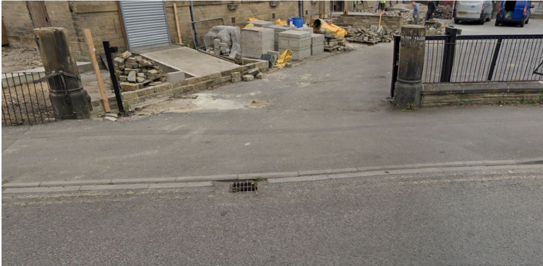
Figure 2 Access to existing car park (Branch Road)
