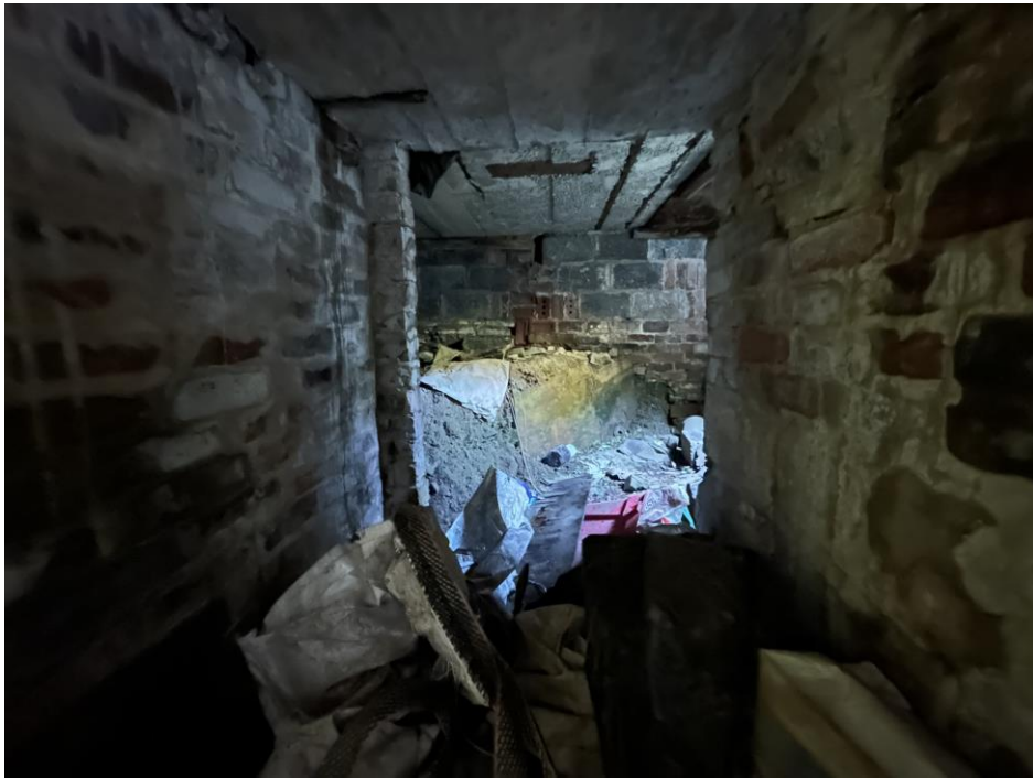
Photograph 2 – Underground area linking the two buildings
