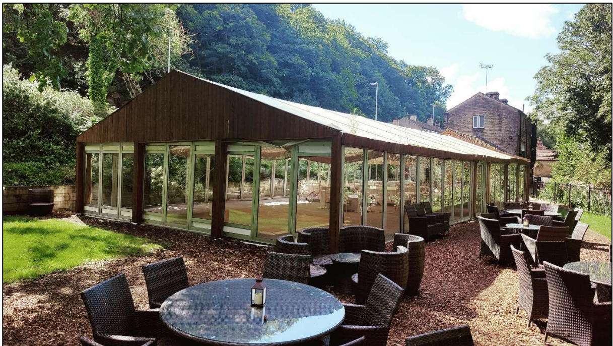
The marquee building forming the subject of this application (northern end view)
