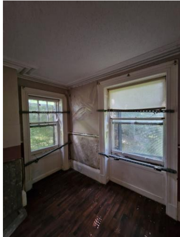
Sash windows with the window (left) having six sections on the upper pane
