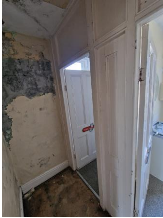
WC and bathroom partition
