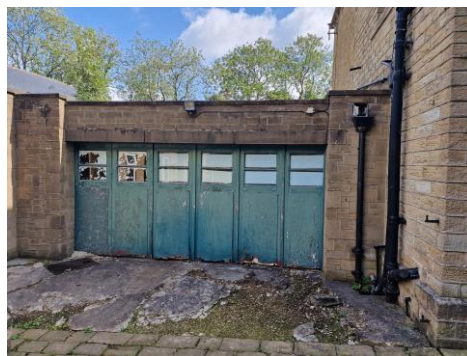
Garage door, buttress walls and coping on flat roof
