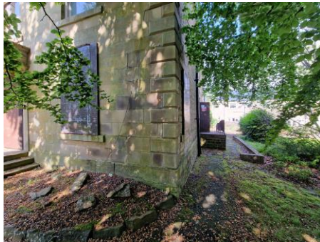
Quoins on the south-east corner facade
