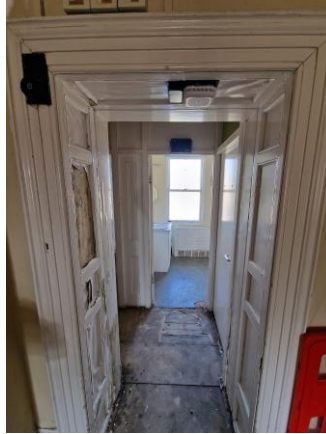
Opening between buildings 1 and 2a/2b
