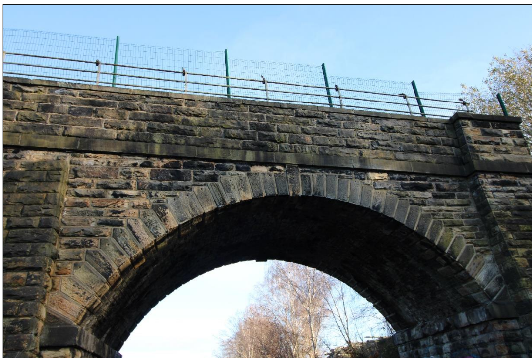
Plate 12: Voussoirs and parapet above eastern span. View facing north-east (IMG_0447)
