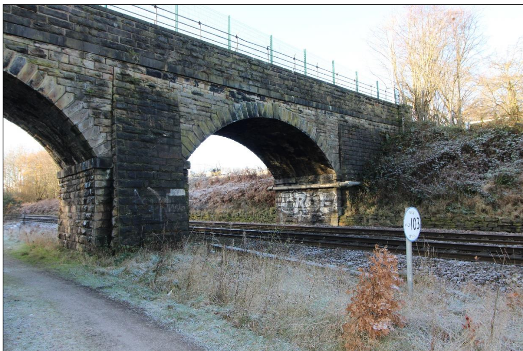
Plate 5: Original western span on northern elevation. View facing west (IMG_0438)
