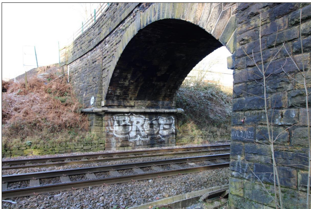
Plate 14: Western abutment beneath western arch. View facing north-west (IMG_0491)
