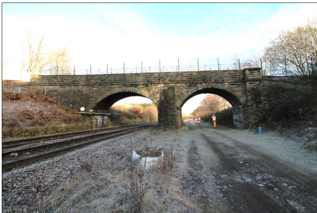
Plate 9: Southern elevation with 1m scale. View facing north-east (IMG_0471)
