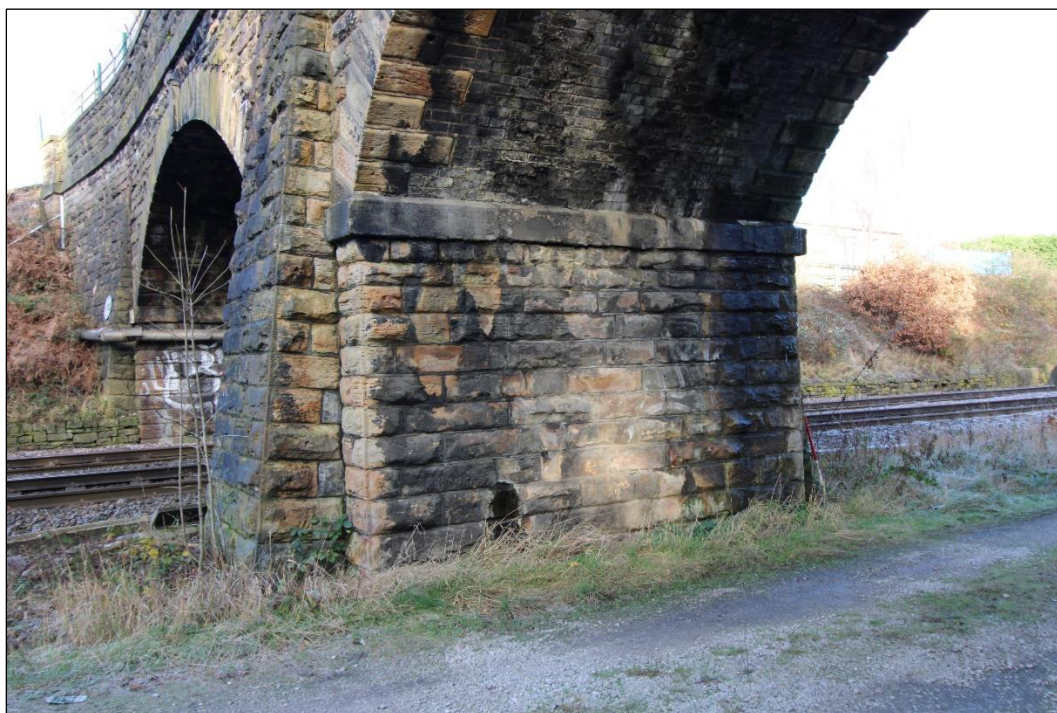
Plate 16: Western abutment of eastern span 2. View facing north-west (IMG_0482)
