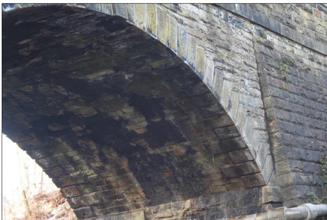
Plate 15: Masonry underside of western arch. View facing west (IMG_9986)
