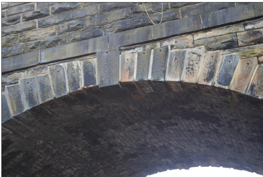
Plate 7: Voussoirs above eastern arch. View facing south (IMG_9992)
