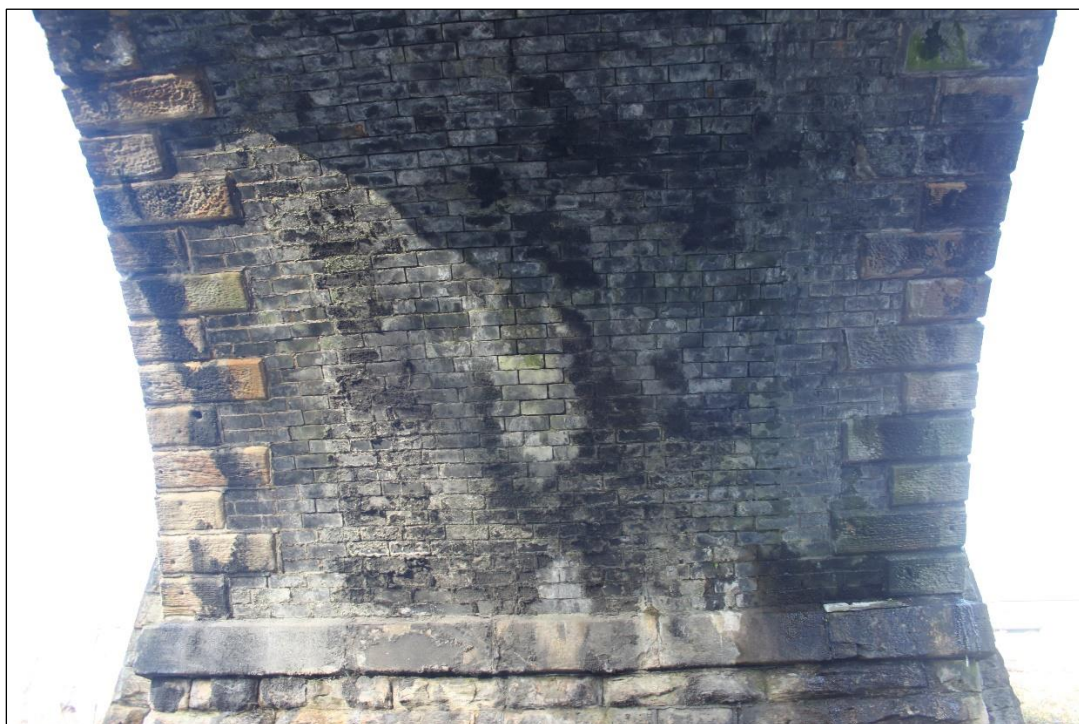
Plate 18: Brick underside of eastern span 2 (western end). View facing north-west (IMG_9965)
