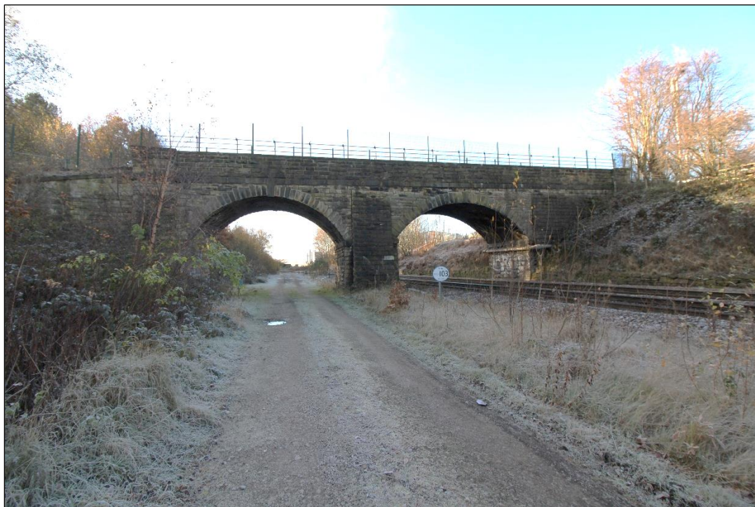
Plate 4: Northern elevation. View facing south-west (IMG_0437)
