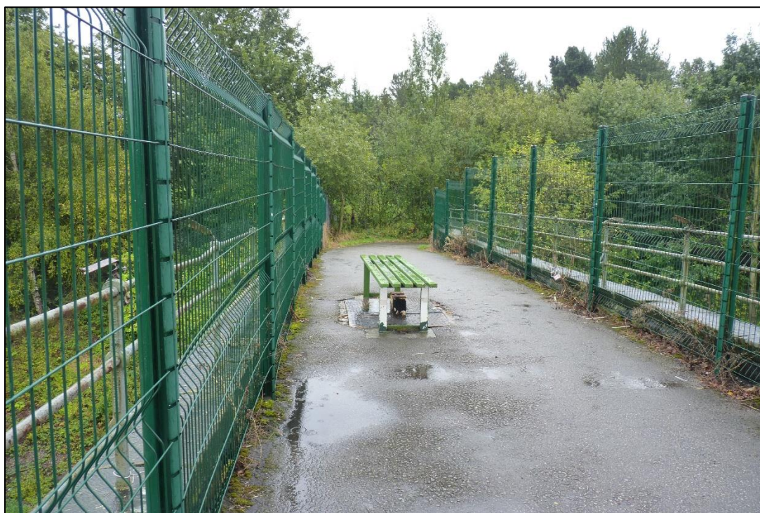
Plate 19: Upper bridge deck, view facing south-east
