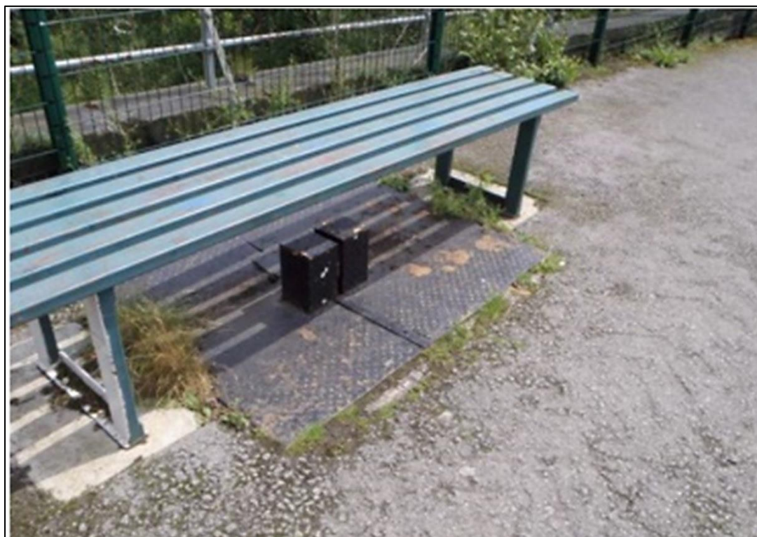
Plate 21: Pedestrian bench above manhole covers. View facing north-east
