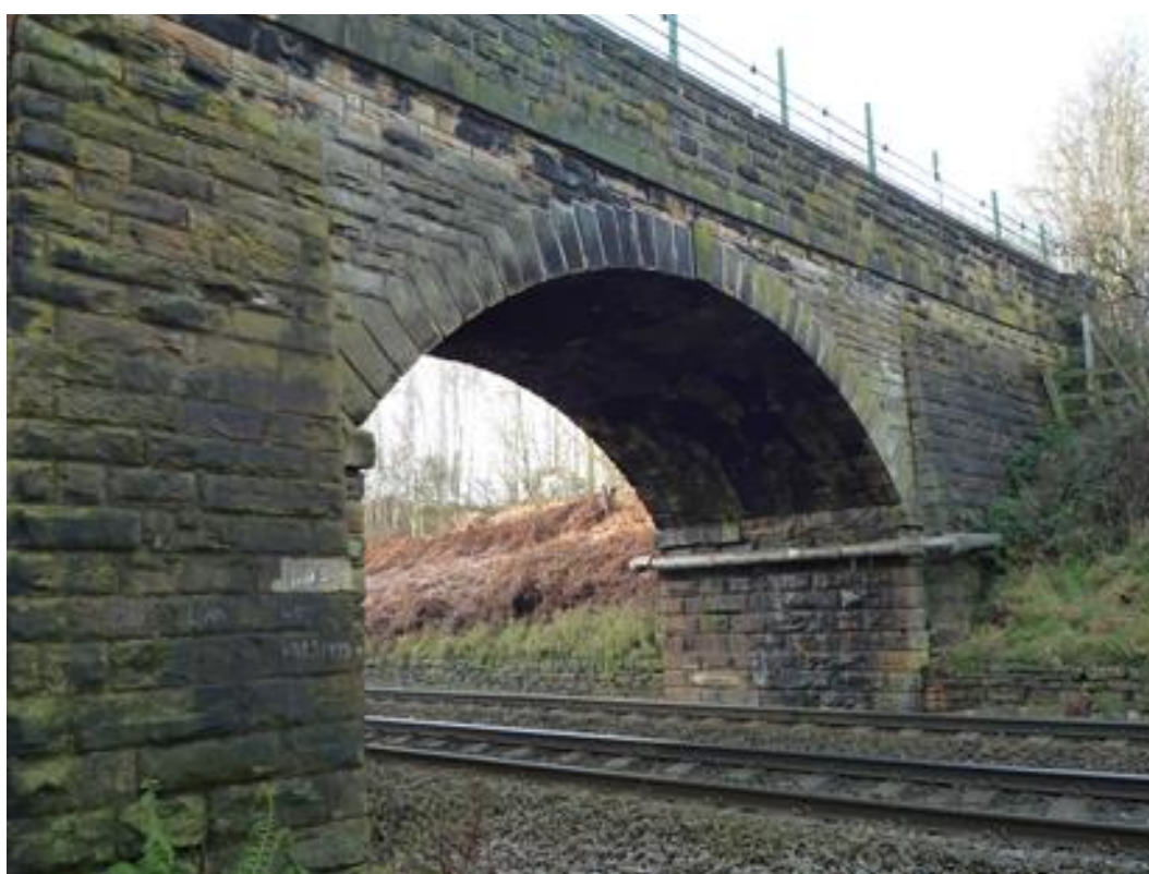
Insert 4-4 Wheatley's (Colliery Lane) Overbridge (MVL3/103), north-eastern elevation, northern span.
