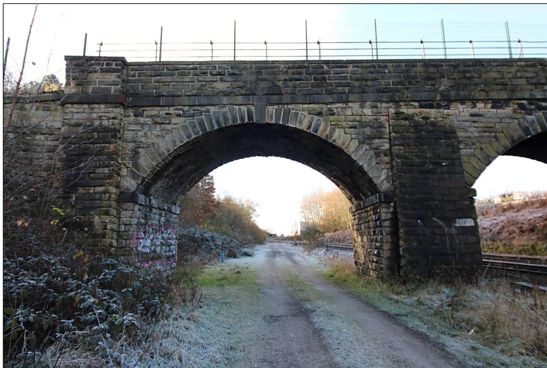
Plate 6: Later eastern span on northern elevation. View facing south-west (IMG_0440)
