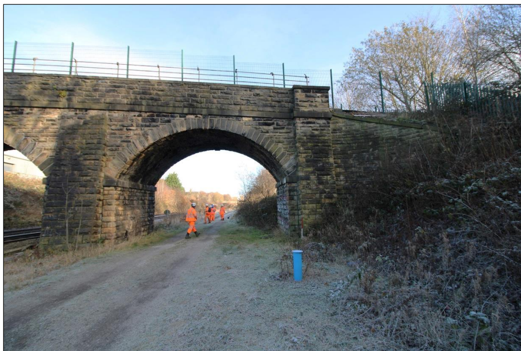
Plate 11: Later eastern span with 1m scale. View facing north-east (IMG_0441)
