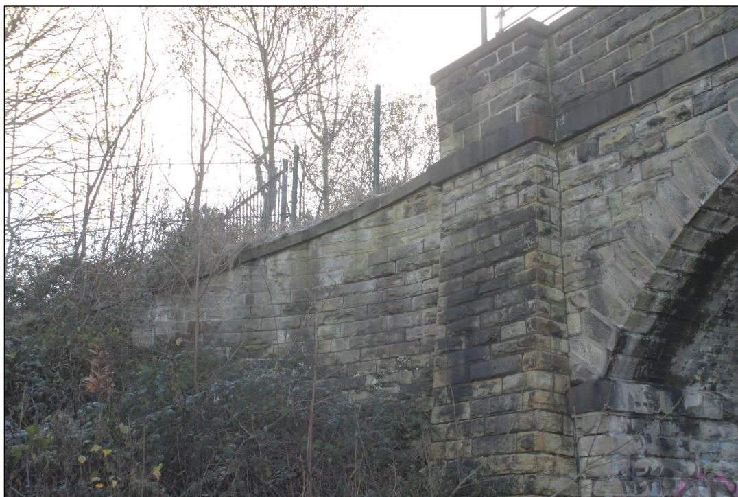
Plate 8: Eastern pilaster and north-facing wing wall. View facing south (IMG_9962)
