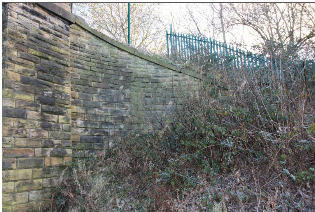
Plate 13: South-facing wing wall. View facing east (IMG_0453)
