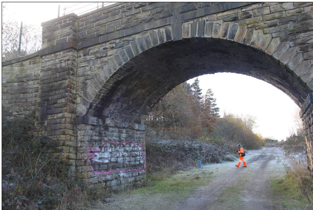
Plate 17: Eastern abutment of eastern span 2. View facing south (IMG_9955)
