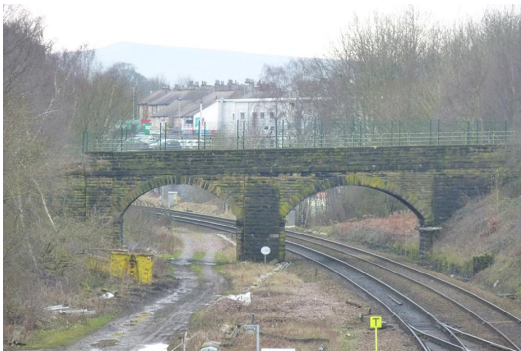
Insert 4-3 Wheatley's (Colliery Lane) Overbridge (MVL3/103), viewed from the north-east.
