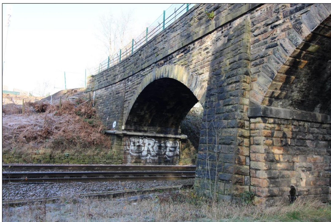
Plate 10: Original western span and angled western end (left). View facing north-west (IMG_0457)
