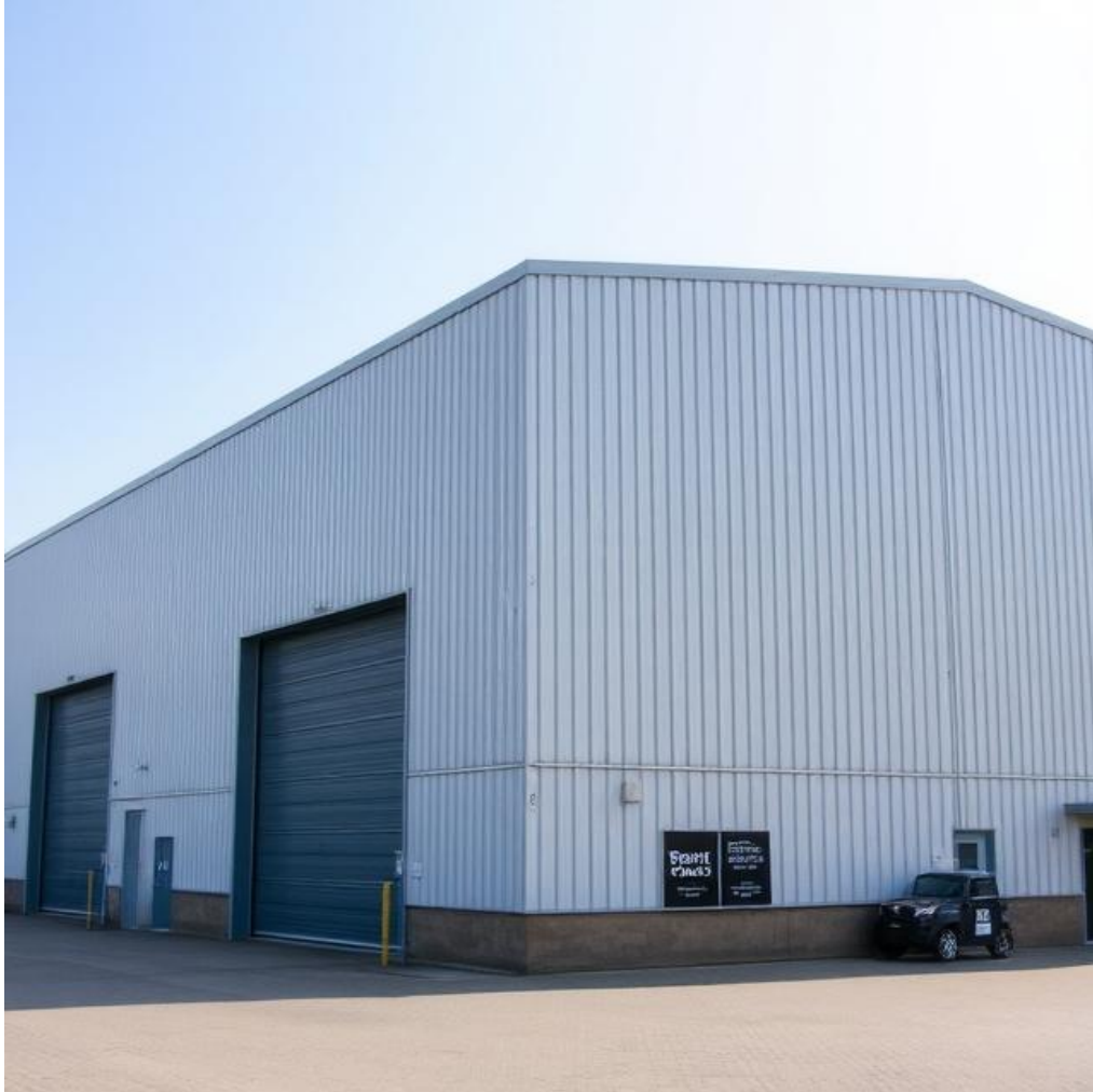
Image 4: Typical example of dark grey cladding
