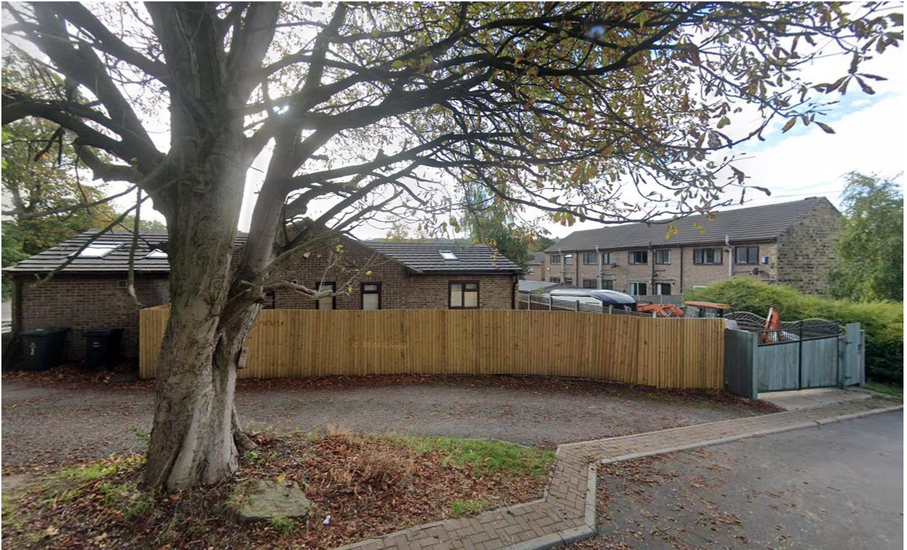
Above: This shows the side elevation of the application property from Savile Mews with the two storey height of the terrace block to the rear within the application property site context.
