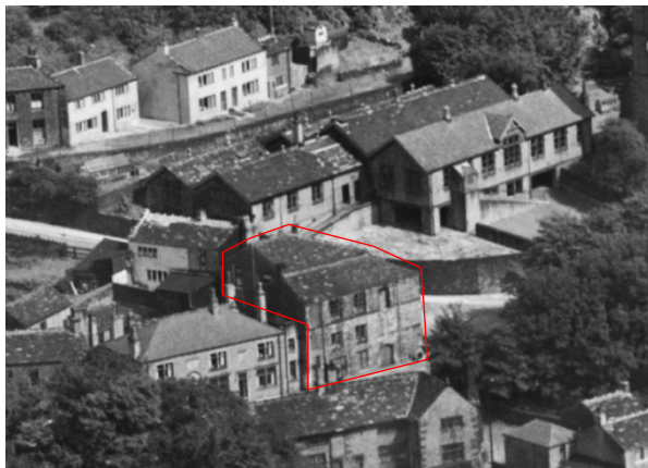
Figure 6: Britain from Above - EAW018228 ENGLAND (1948). Upper Mill and environs, Slaithwaite, 1948.
