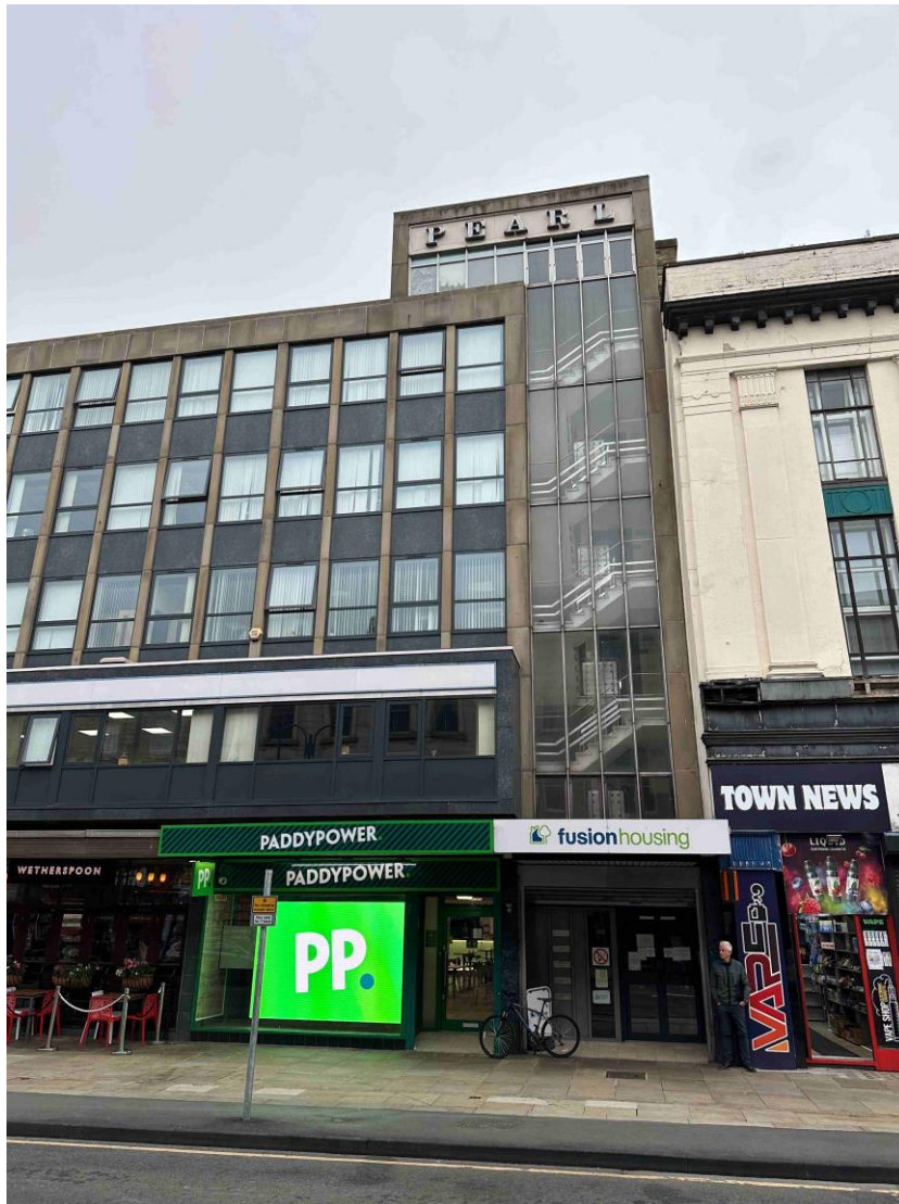
Photograph 2 – Entrance to the Upper Floors of Pearl House
