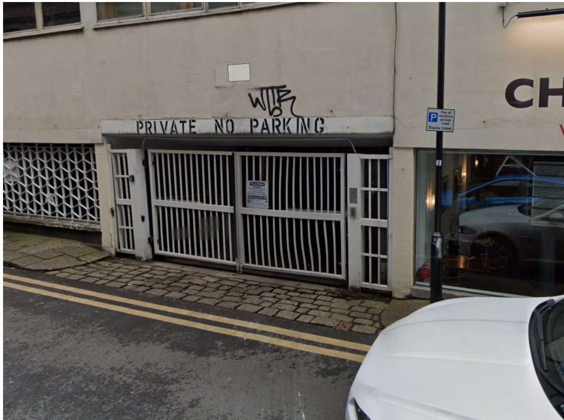
Photograph 3 – Rear Vehicle Entrance off Wood Street.
