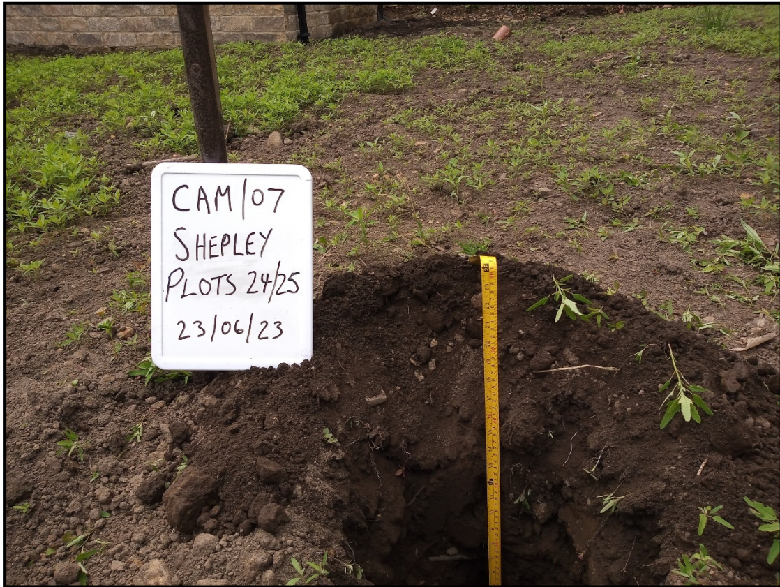
Plots 24/25: Clean cover validation pit, tube removed, 0.6m depth achieved.
