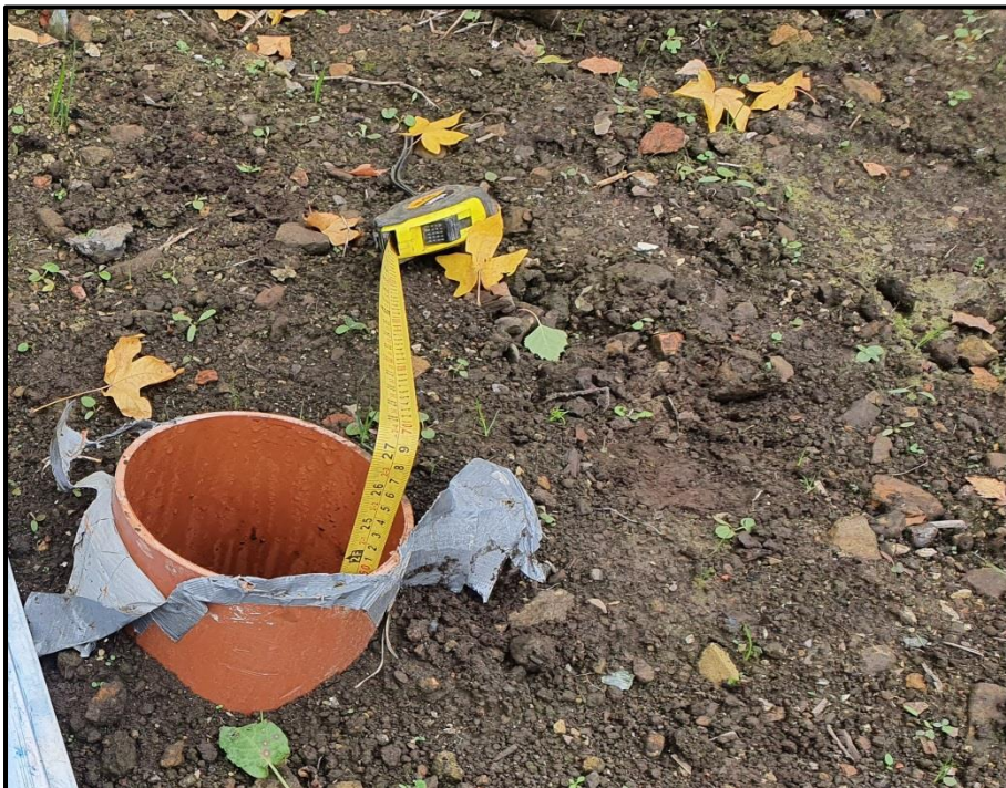
Plot 12: Depth measured in tube left by groundworker. Over 0.6m in cover.
