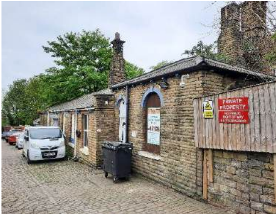
Photograph 1: Buildings B1a and B1b.
