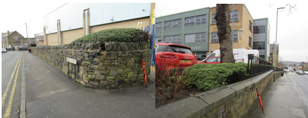
Low stone walls to Church Street, Grove Street and High Street on South, East and North Elevations
