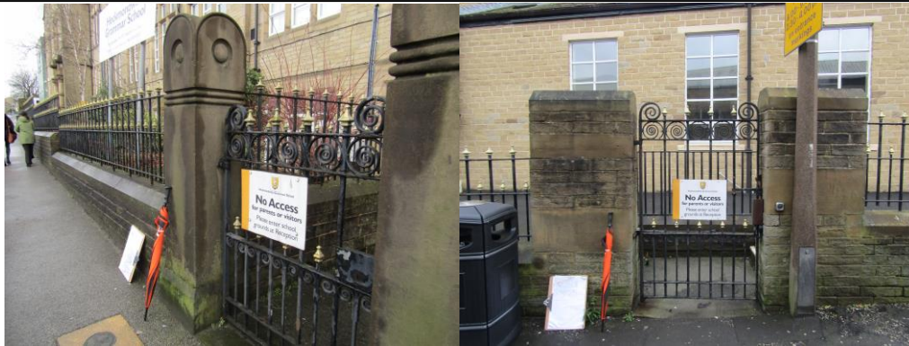
Original ornate pedestrian gates to High Street and North Street on North and West elevations
