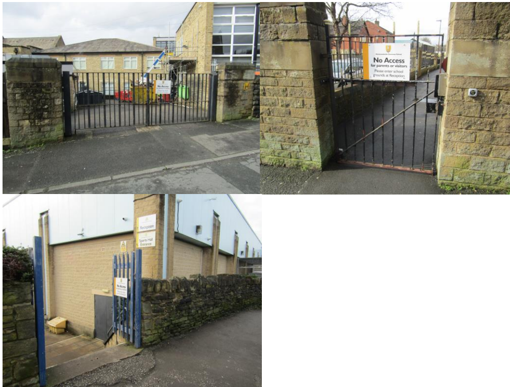
None original vehicular/pedestrian gates to Church Street and Grove Street on South and East elevations.
