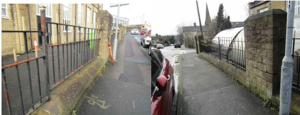
Low boundary stone wall with standard railings to North Street and Church Street on West and South elevations
