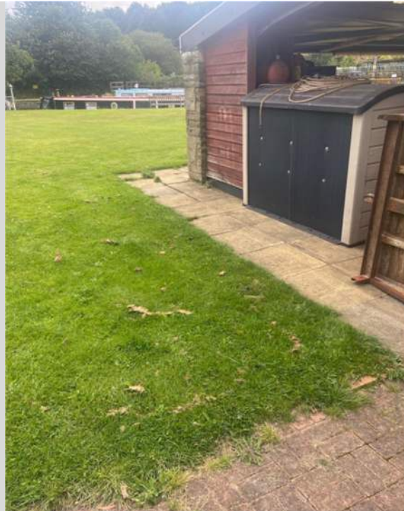
13. Northwest end of enclosure, from north. This is where the proposed workshop as detailed in the planning application will be located.
