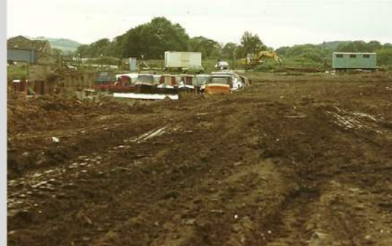
12. Arisings used to infill drainage ditch and lagoon to rear of dry dock, after new culvert installed
