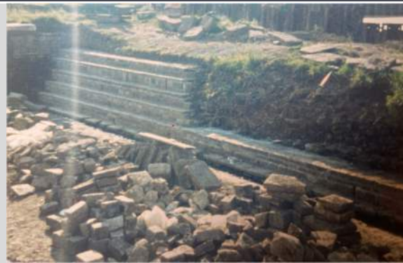
13. February 1987 rebuilding of walls with original stone.
