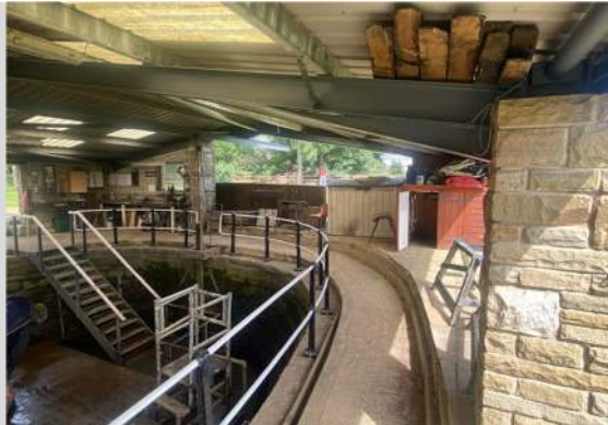
7. Northeast end of dock from inside enclosure.
