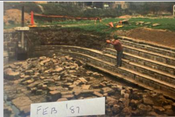
14. February 1987 rebuilding of walls with original stone.
