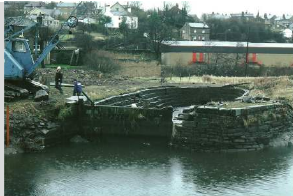
7. December 1986, excavation of new mooring basin started adjacent to the dry dock.
