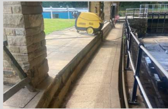
8. Southeast wall of dry dock from northeast.
