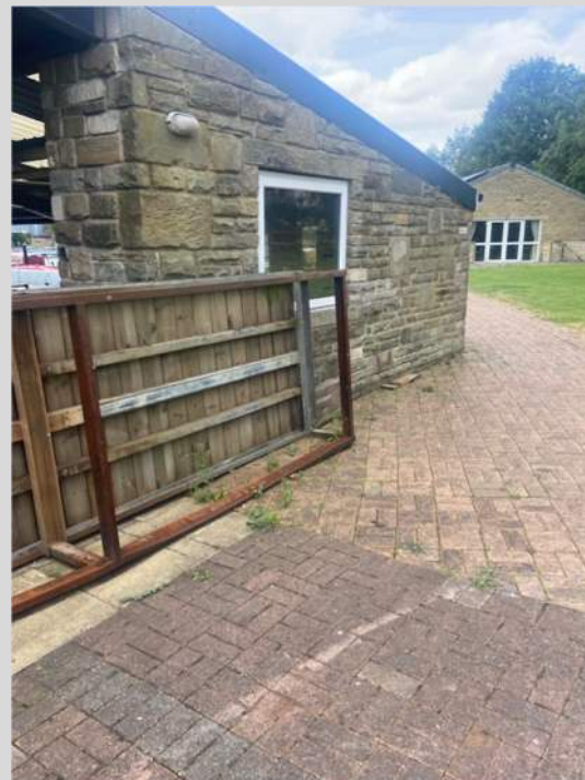
14. Northwest end of enclosure, from east. This wall will remain unchanged.
