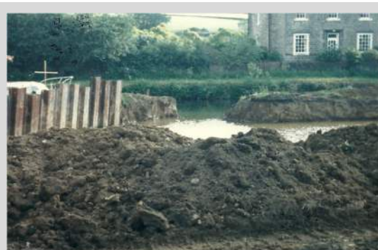
10. Arisings from basin excavation
