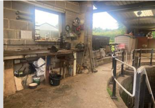
10. Northeast wall of enclosure from inside.
