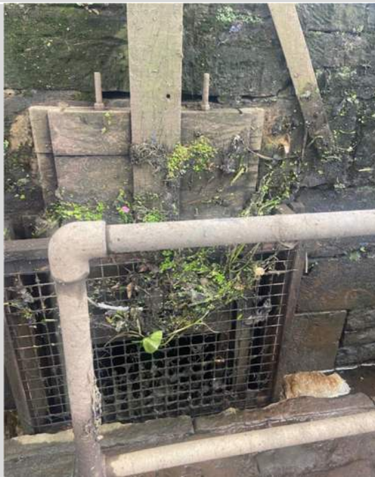
11. Sluice gate at northeast end of dry dock. The drainage ditch and lagoon have been replaced with a culvert that feeds directly into the River Calder.
