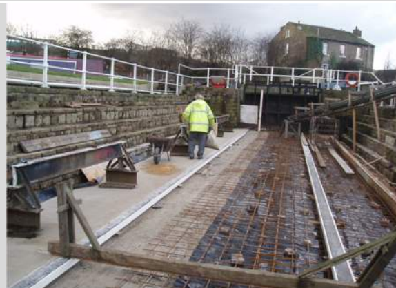
17. Reinforced concrete laid over original stonework at base of dry dock.
