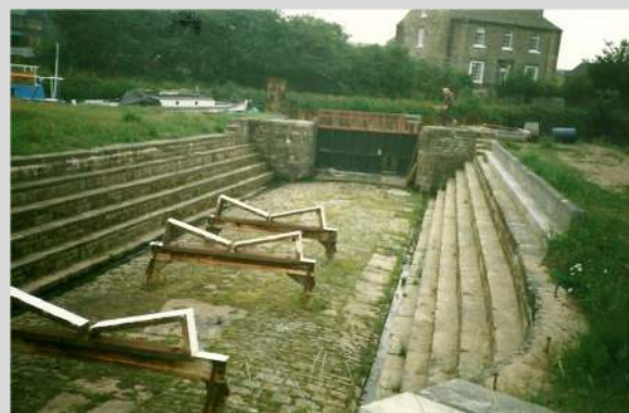
15. July 1988, new gate and boat supports installed.
