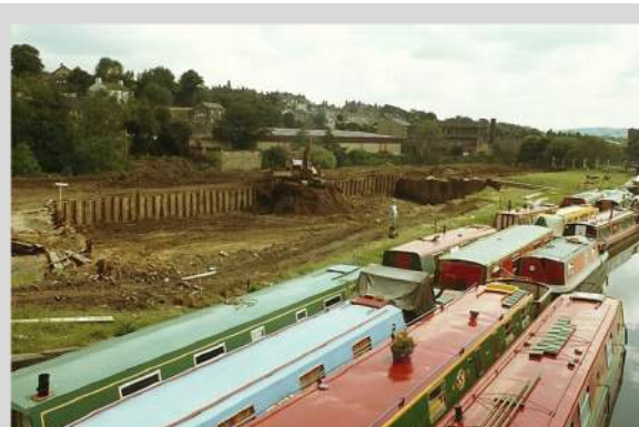
8. Basin excavations continued
