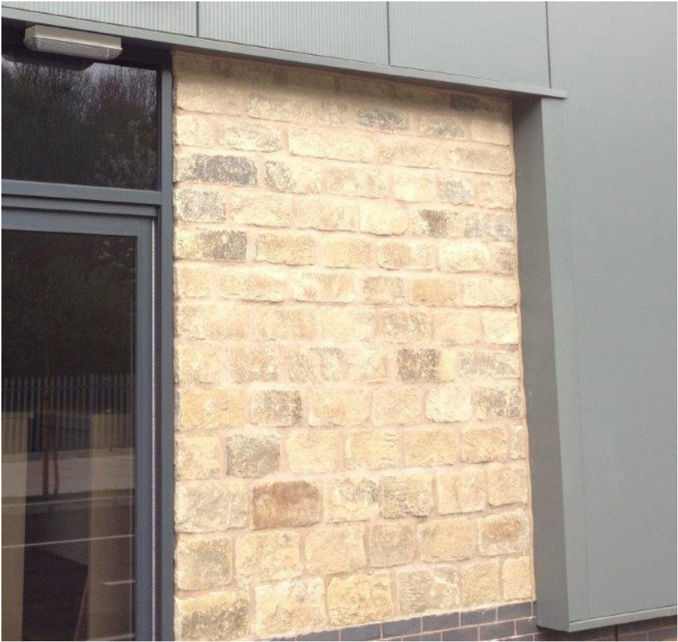
Above - Sandstone masonry
