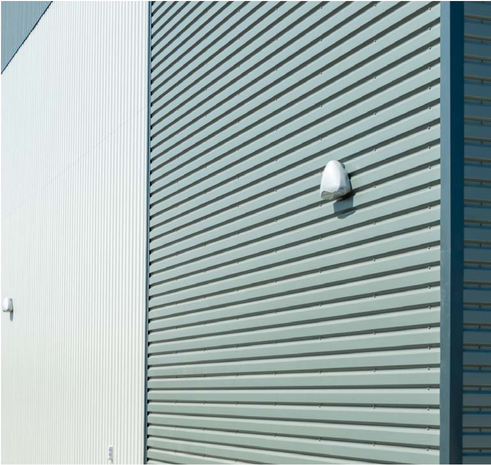
Above - Horizontal profile built up cladding
