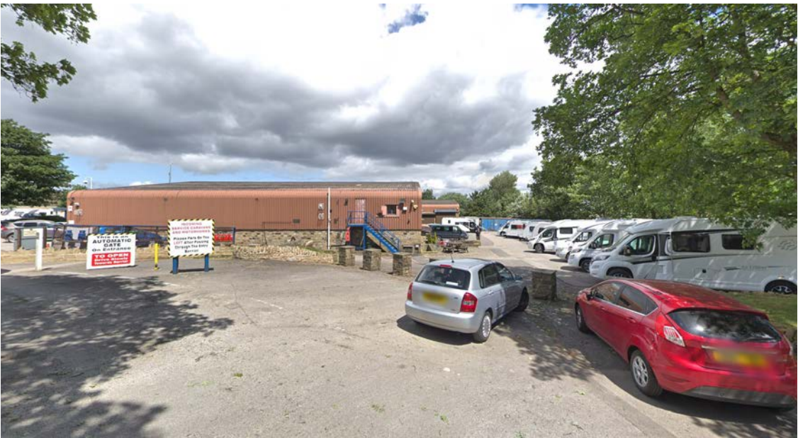
2 - Existing sales office and workshop building
