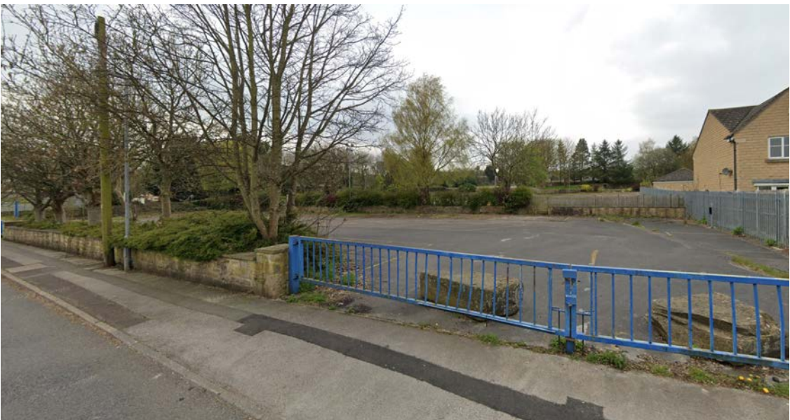
3 - Existing access on Crosland Hill Road (lowest point)
