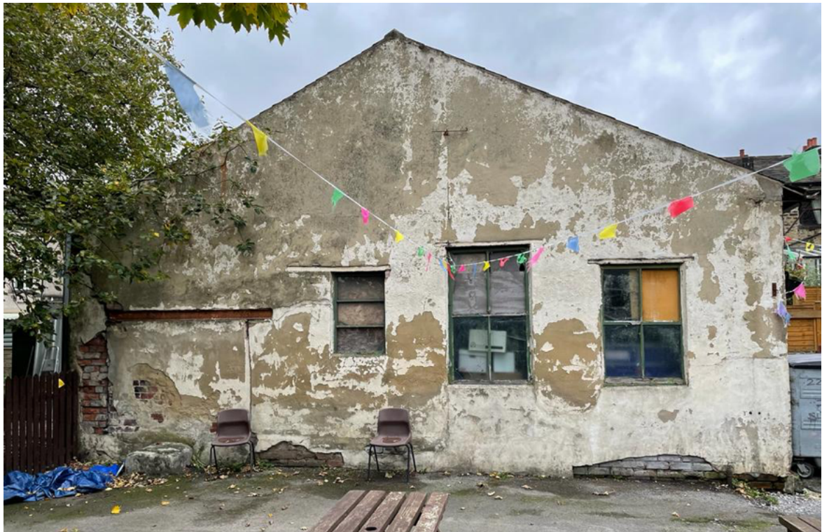
North elevation 4 of 37
