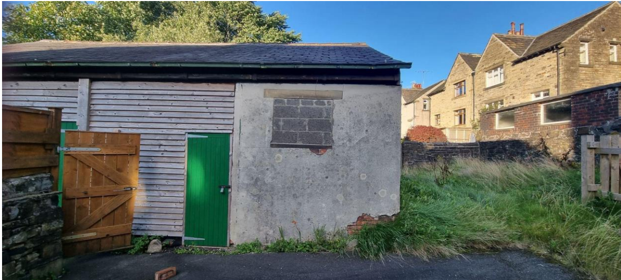
Figure 1-2: Barn on the site
