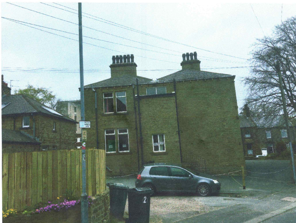
View of the rear elevation
