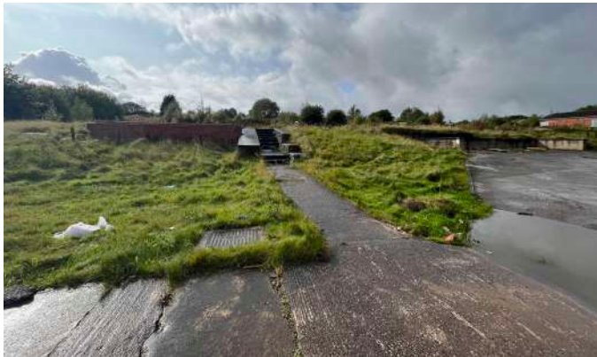
1. View of demolished building footings associated with the previous use.
