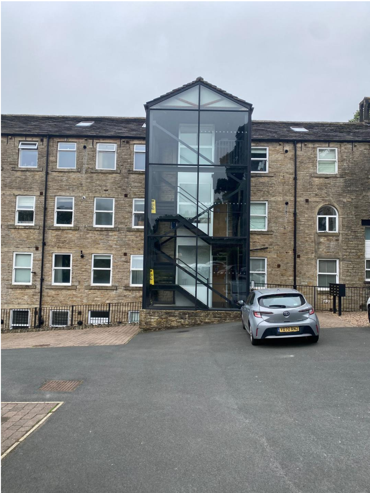
Figure 3 A photograph of the front elevation of the main mill building adjoining the pump house
