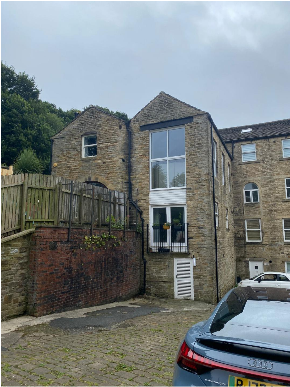
Figure 4 A photograph showing the rear gable of 110 underbank old road and the adjoining neighbouring property with original largescale glazing
