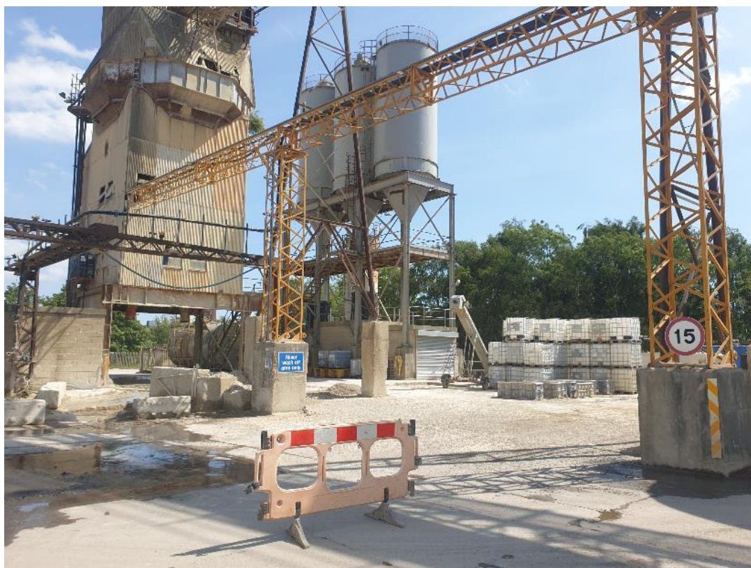
Photograph 7: Concrete silos at northeastern end of the site, facing northeast.
