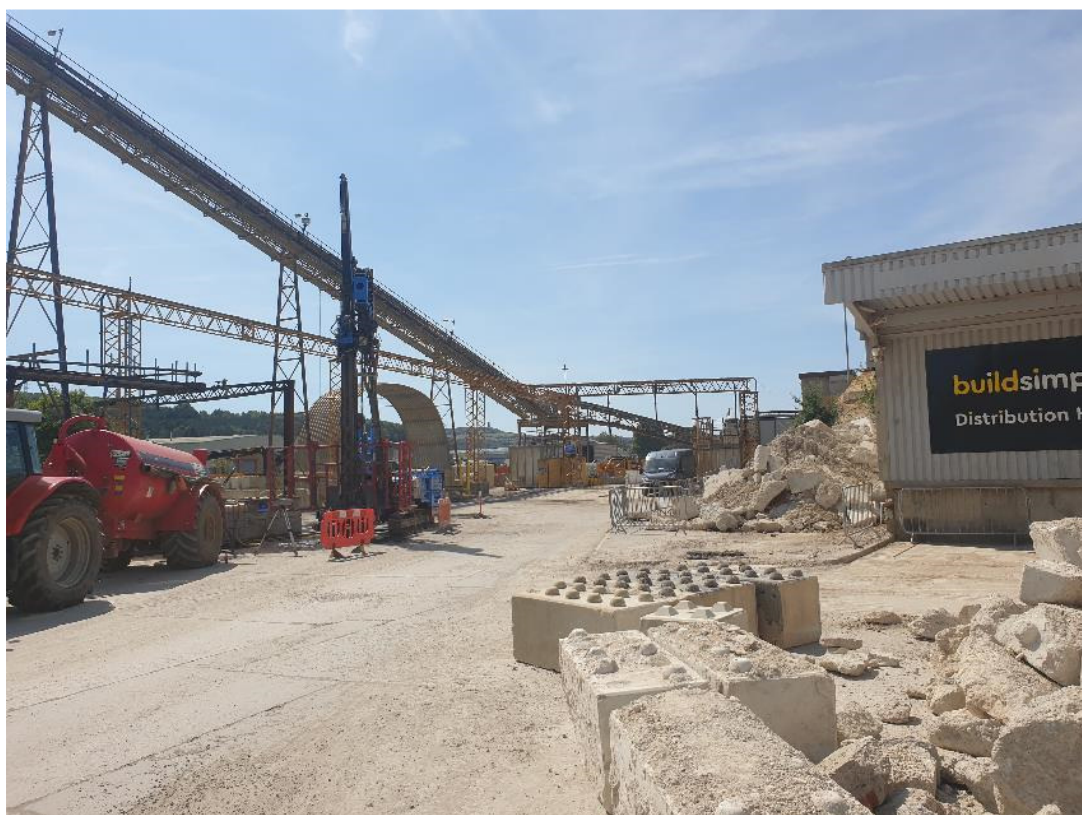
Photograph 4: Infrastructure associated with the former concrete plant at the centre of the site.
