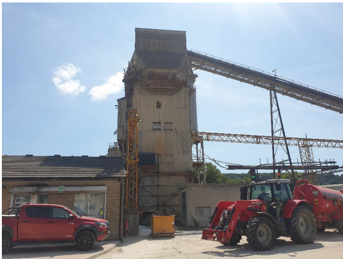
Photograph 6: Mixing tower associated with the former concrete plant at northern end of the site.
