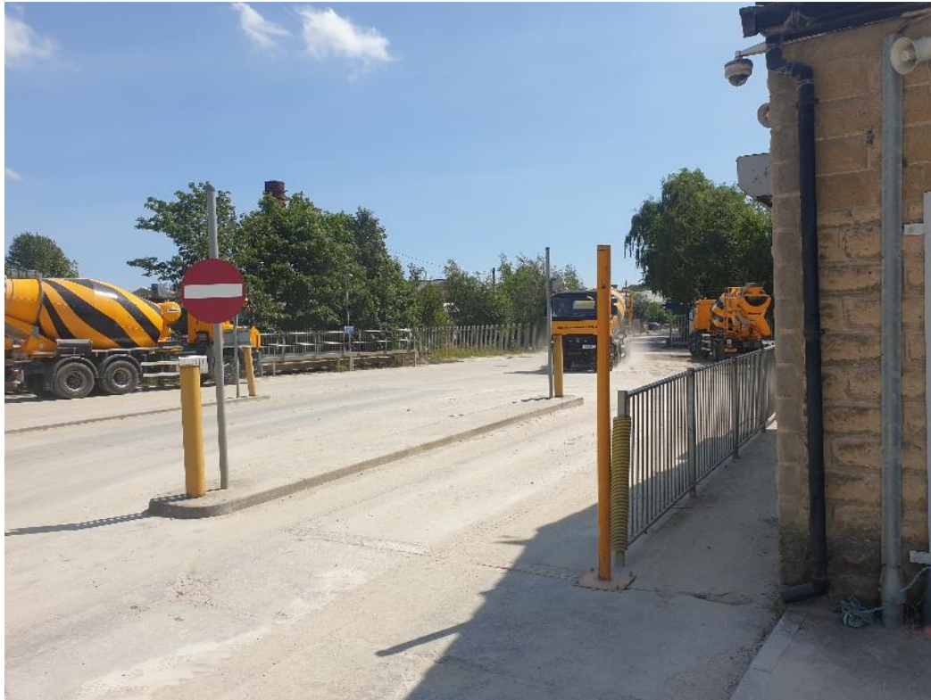
Photograph 1: Entrance off Red Doles Lane to the northeast of the development boundary.
