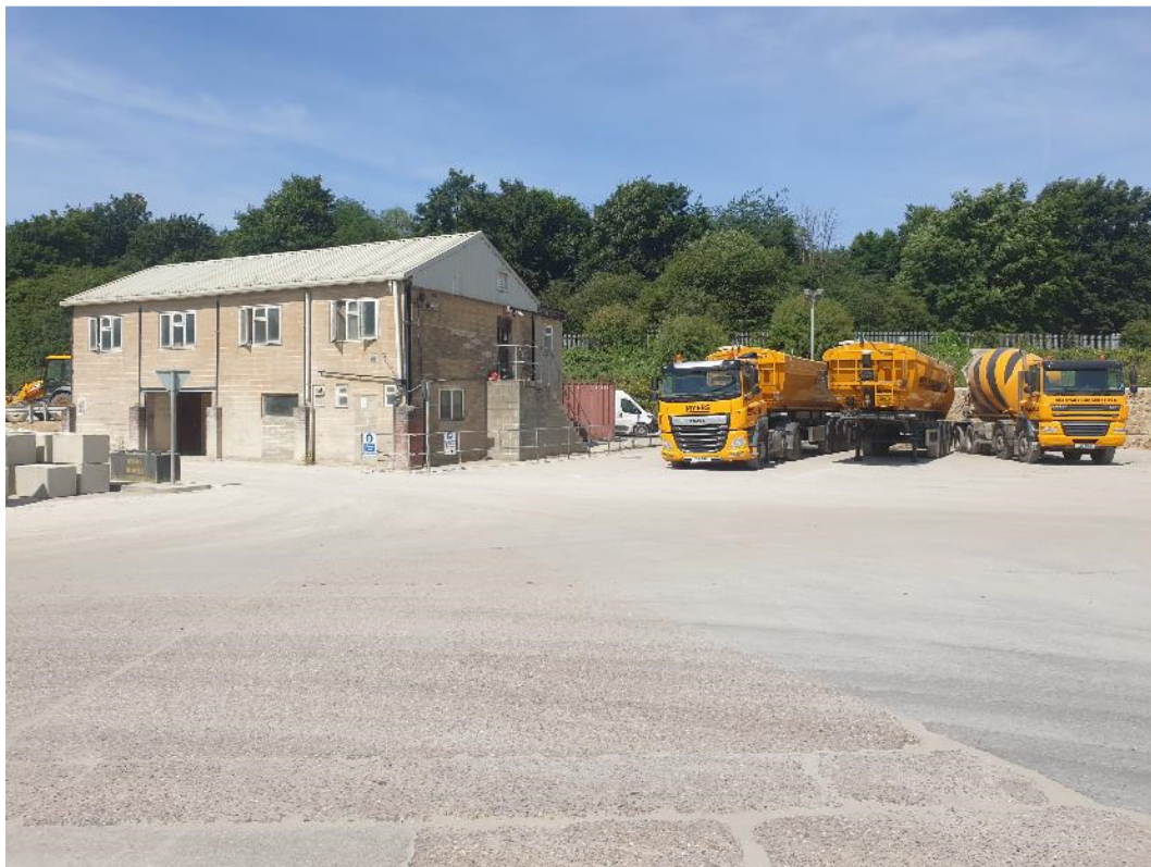
Photograph 2: Two storey building at northern boundary of the site.
