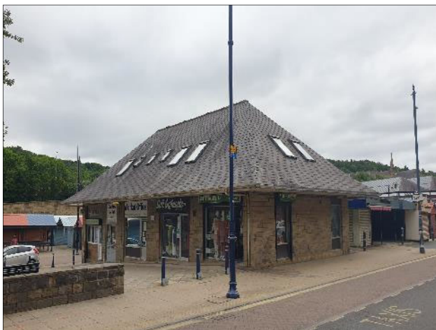
Plate 11. External view of the existing market office in the north-eastern corner of the Site.
