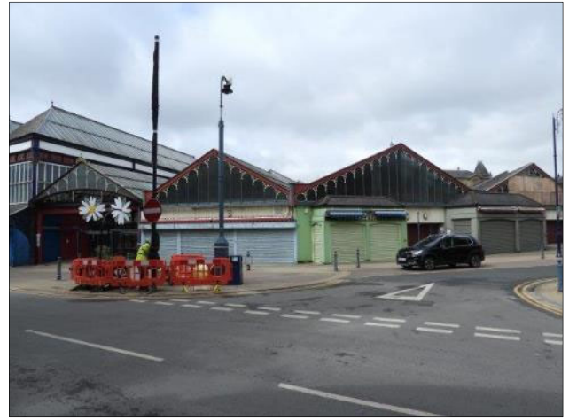
Plate 2. View from Whitehall Way on the eastern side of the Site looking south-west towards the lower level market hall, and surrounding hard standing.
