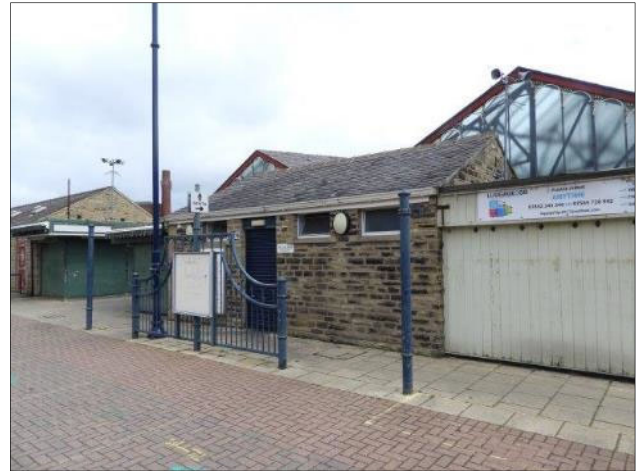
Plate 4. Gents toilet block .and adjacent permanent trader stalls.
