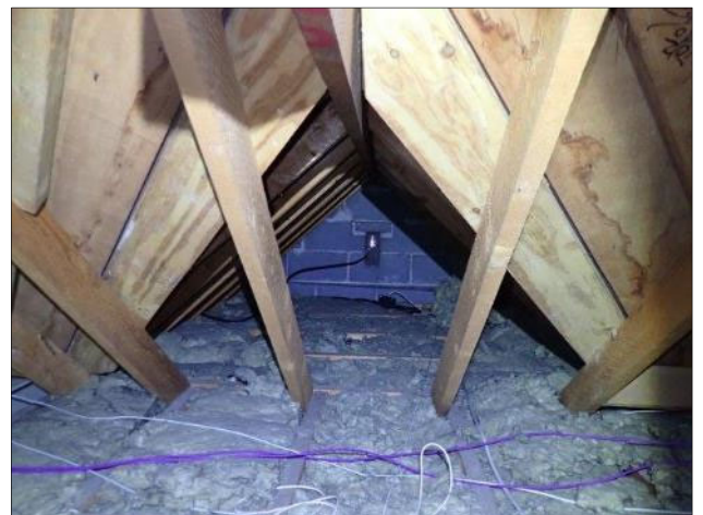
Plate 12. The market office; view within the internal loft void
