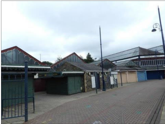
Plate 3. Ladies toilet block in the centre of the Site
