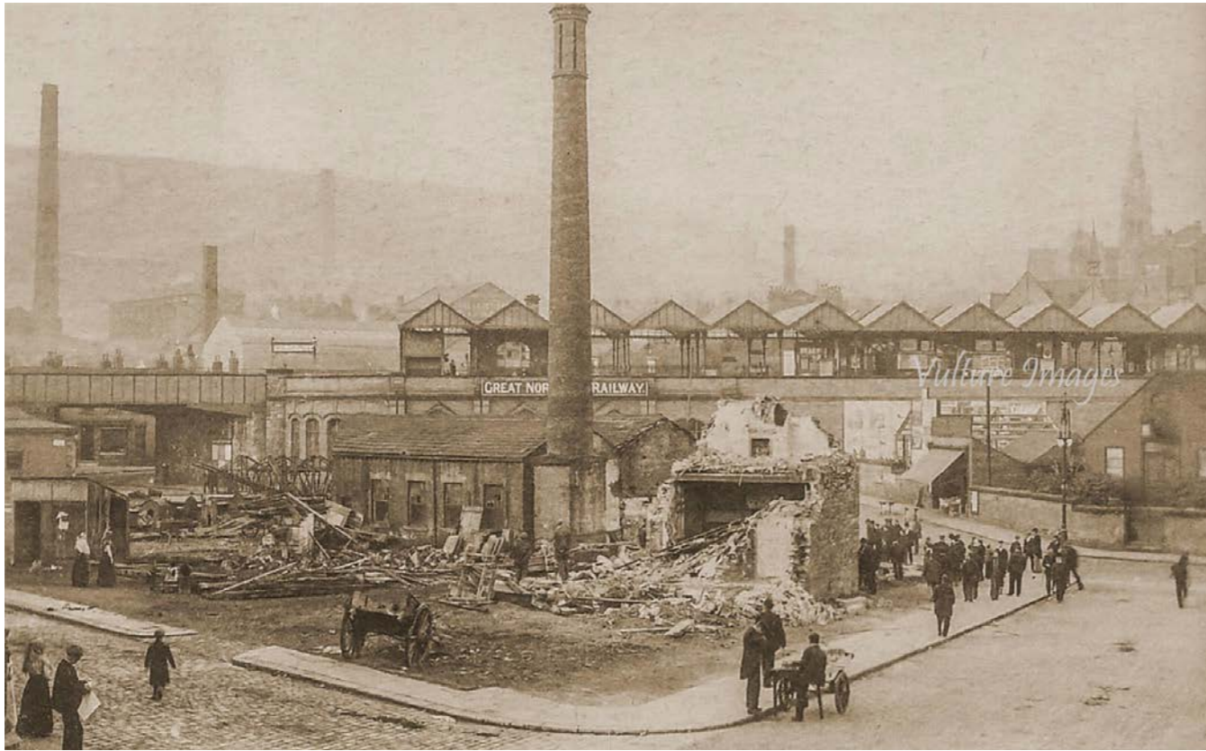
Figure 8: Site clearance on Foundry Street in advance of the construction of the new Market Hall. [Photograph]. At: Mirfield Archive ( https://features.mirfieldarchive.org/dewsbury-in-old-pictures-postcards-gallery )
