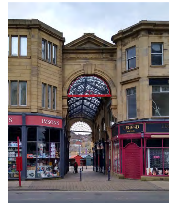
Figure 2.3.12 View through Kingsway Arcade (BDP 2021)
