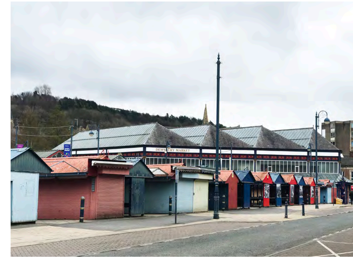
Figure 2.3.9 Outdoor Market and Market Hall from Foundry Street (BDP 2021)
