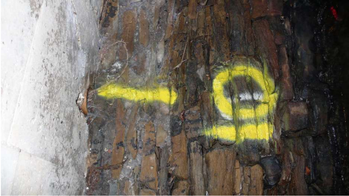
Photograph 7 10.0m LHS 4" drainpipe through concrete soffit.
