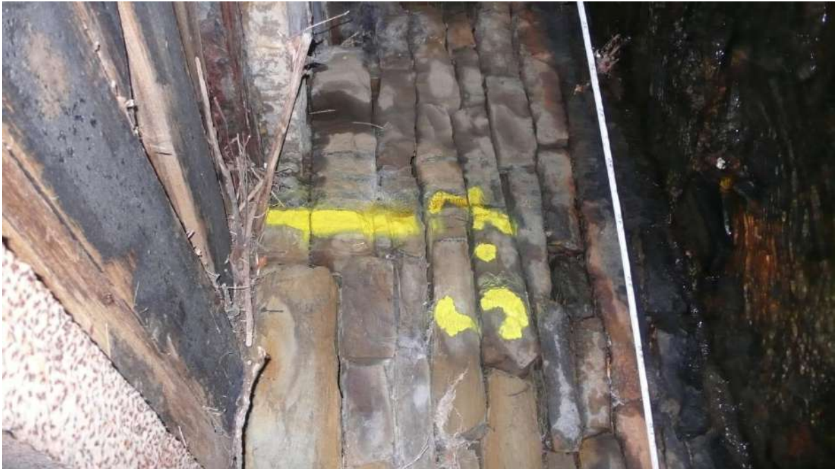
Photograph 5 5.7m LHS second RSJ and timber soffit formwork.
