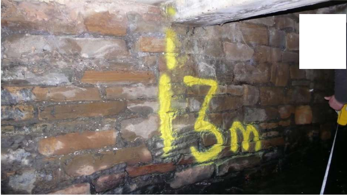
Photograph 11 13.0m LHS concrete beam.
