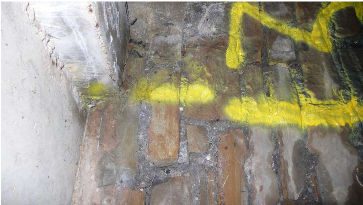
Photograph 12 13.0m LHS close-up of bearing of in-situ beam onto stone wall.
