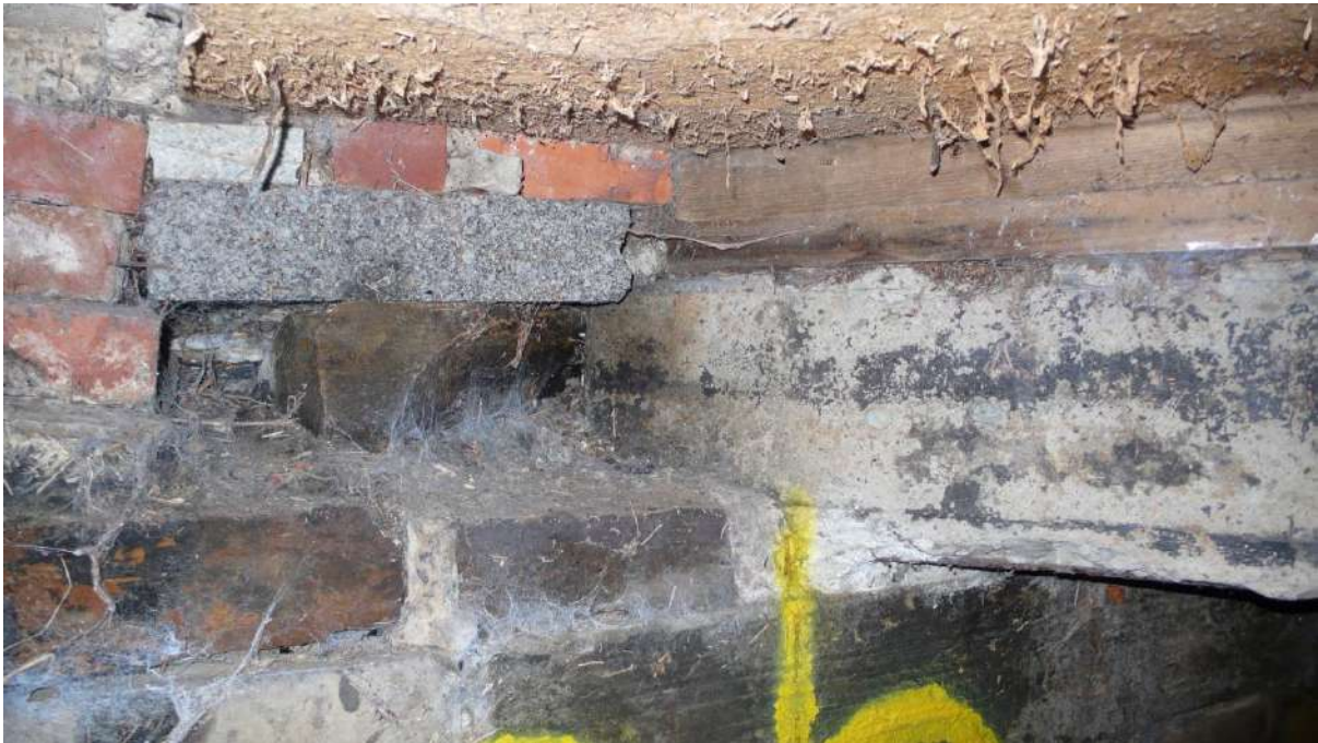
Photograph 29 22m RHS close-up of picture 28 above
