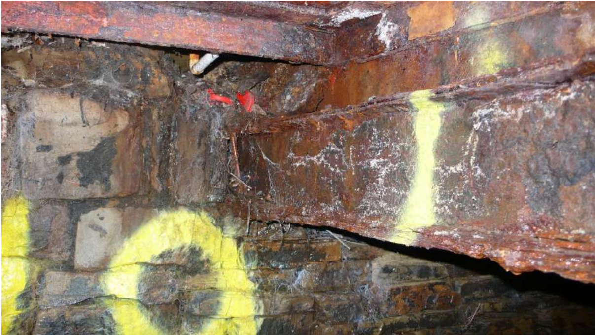
Photograph 31 19m RHS close-up of picture 30 above
