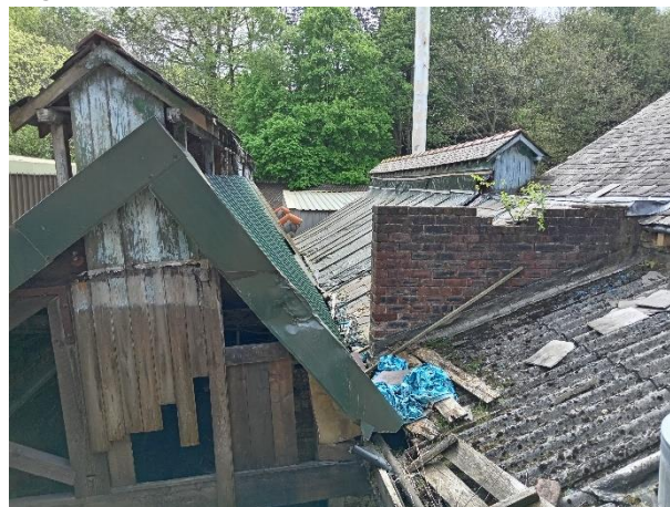
Figure 23 Limited views of B6 &7
