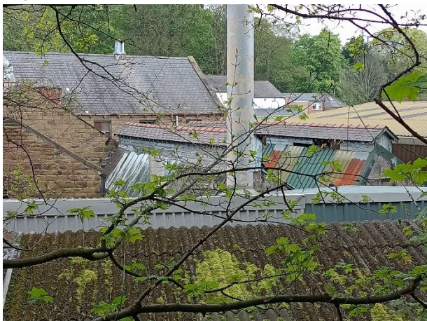
Figure 22 Limited views of B6 &7
