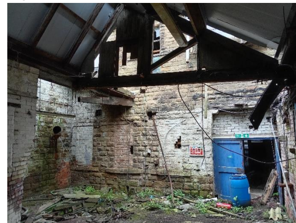
Figure 24 Internal views of B6 & 7
