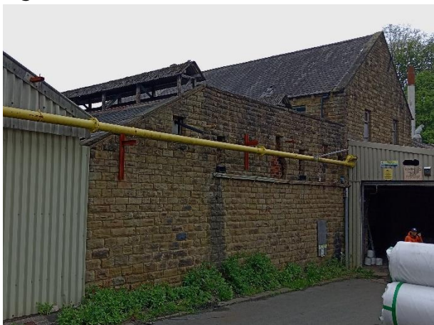
Figure 25 View of B8 & 9
