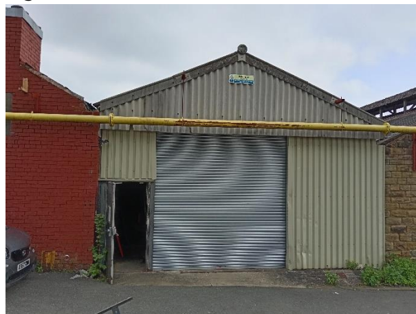
Figure 26 View of B9
