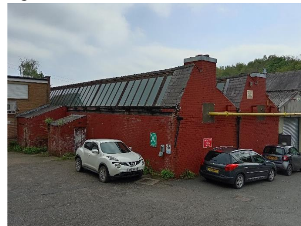
Figure 27 View of B10
