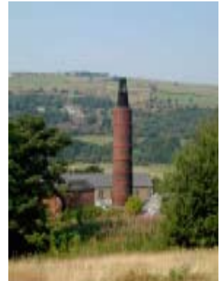
Brick was a good material for chimney construction
