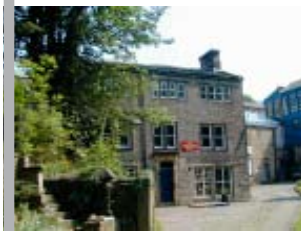
Black Rock House a Grade 2 listed building
