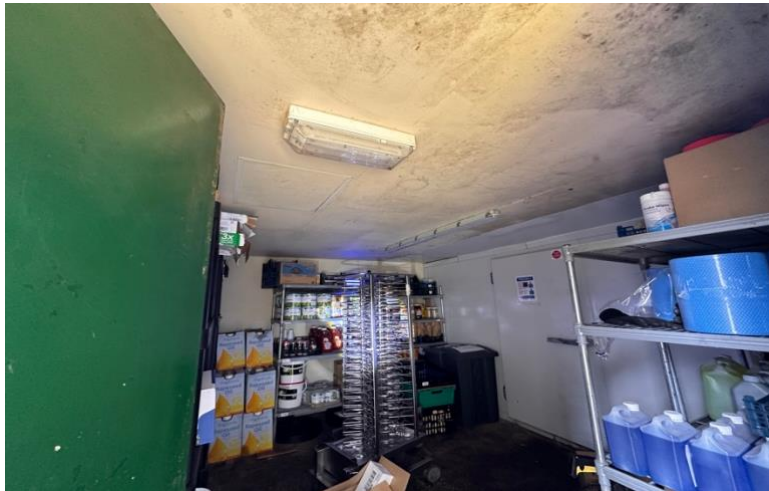
Image 35: Internal space of B2
