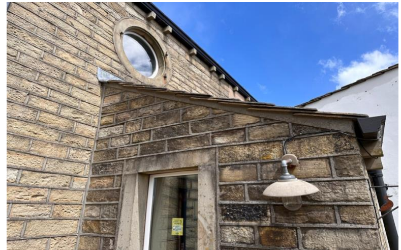
Image 20: In tacked brick and mortar along the northeastern elevation of B1
