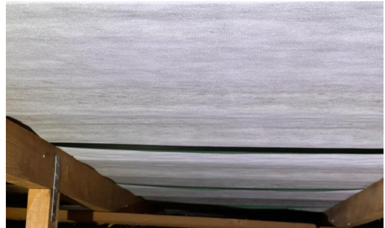
Image 26: Area of water damage to the breathable membrane within L2
