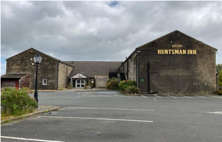
Image 5: Southwestern elevation of B1
