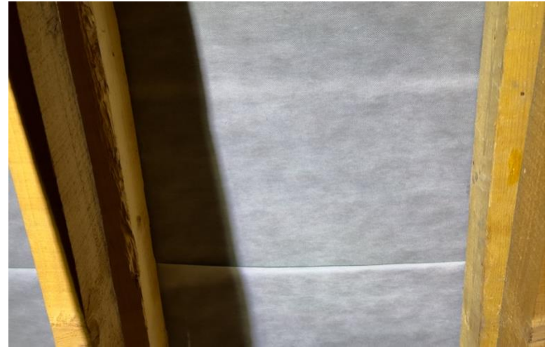
Image 22: Breathable membrane lining with L1
