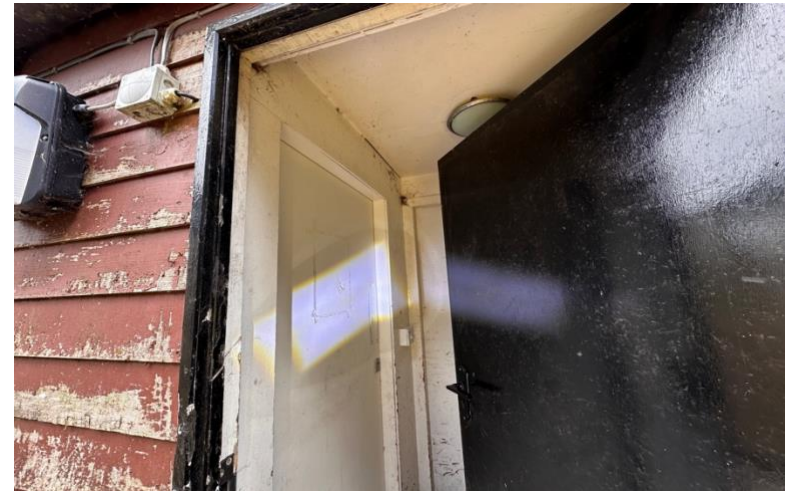
Image 36: Internal space of B2
