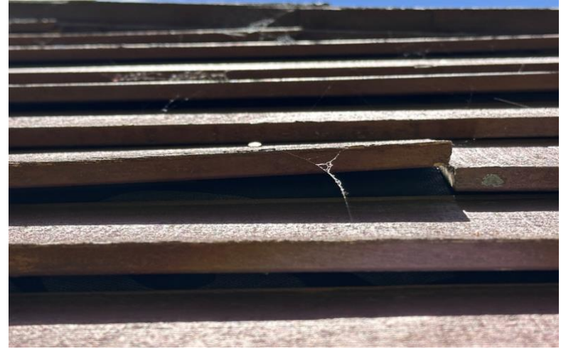
Image 34: Gaps under the lifted wooden panelling on B2
