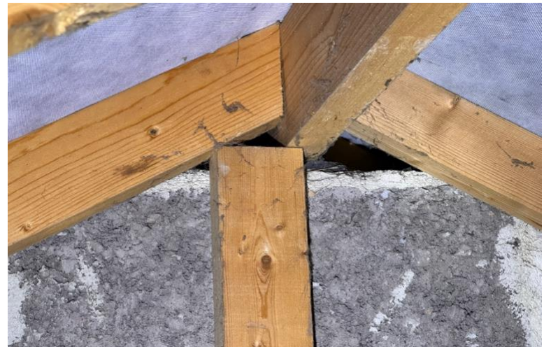
Image 22: Breathable membrane lining with L1
