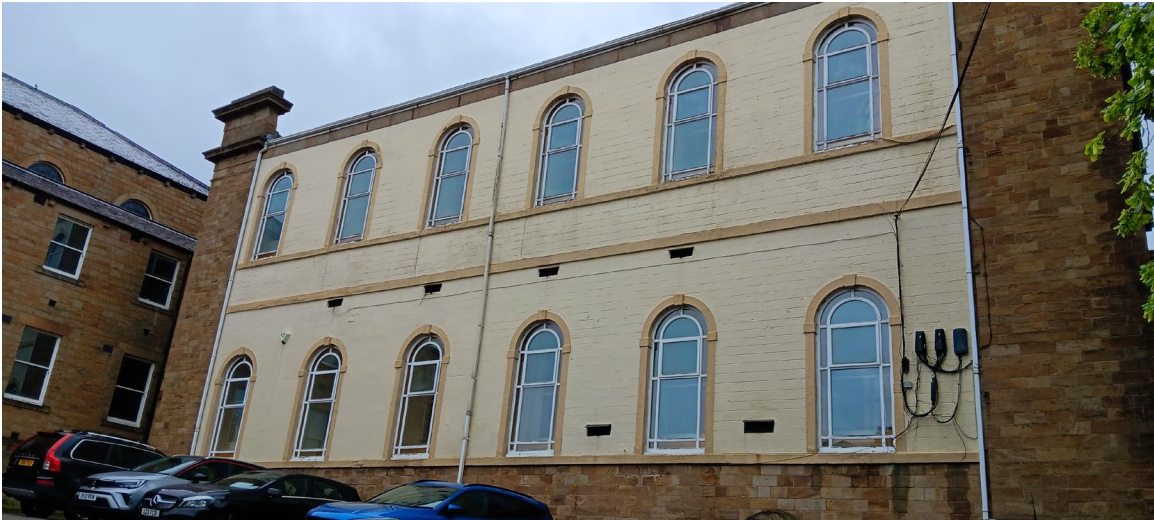
Fig.2 – Chapel lane Elevation – with painted stonework
