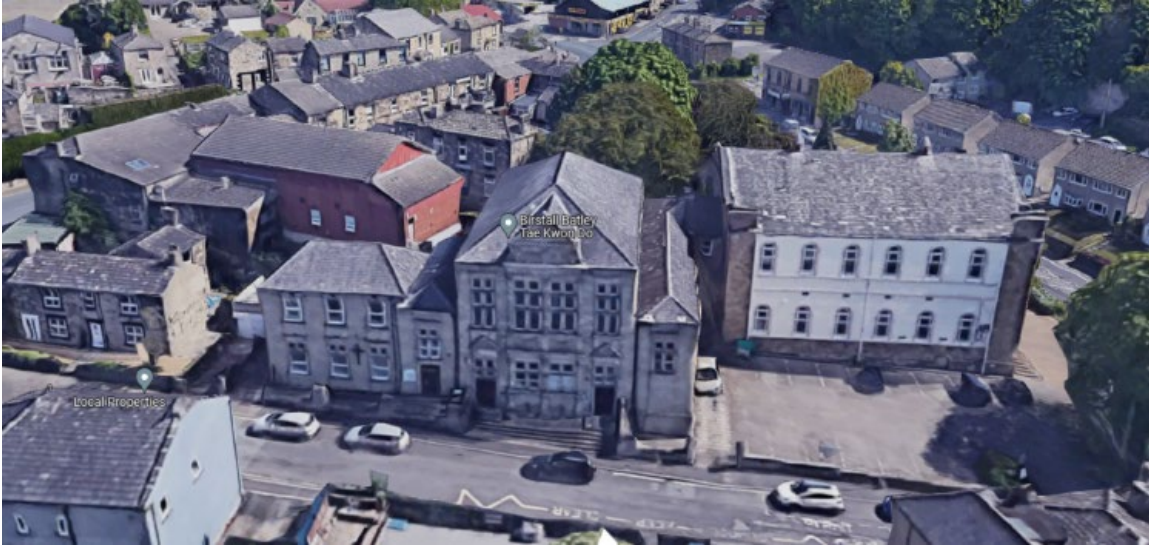
Fig.2 – Front view of building and surrounding properties
