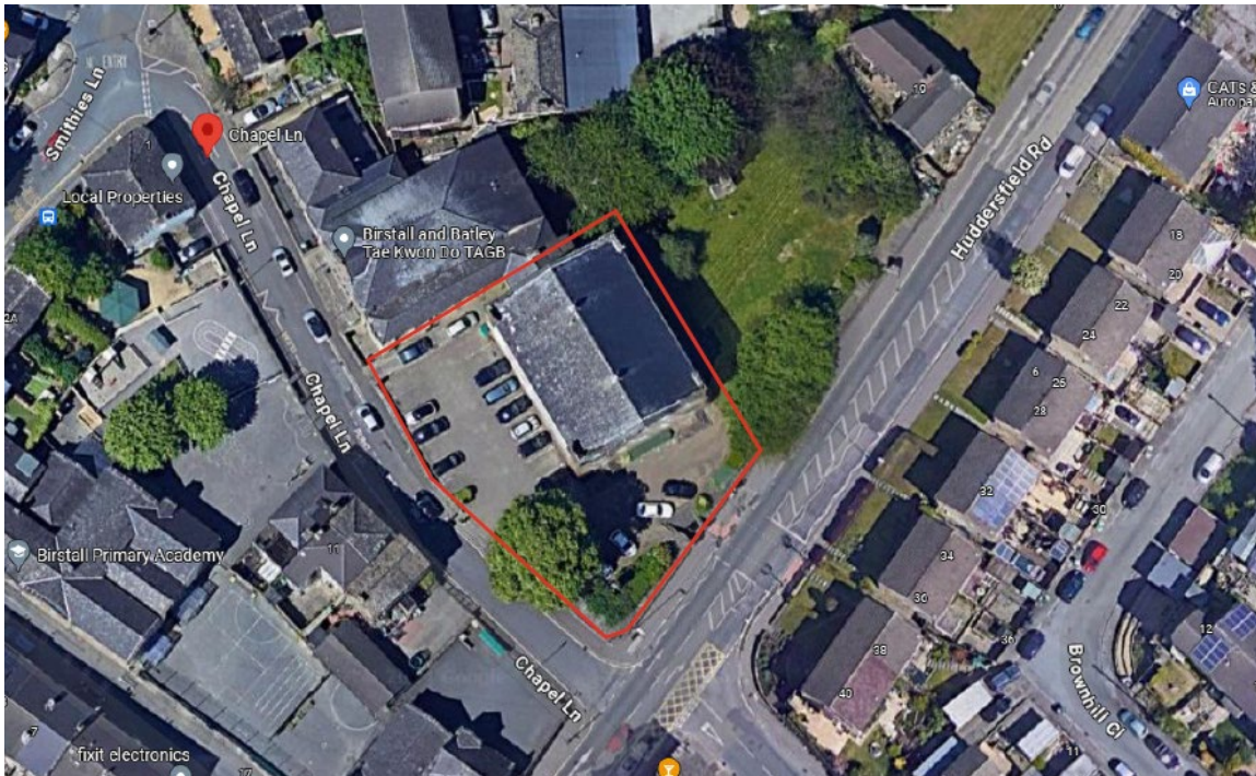
Fig.1 – Ariel view of site
