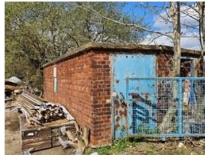
B1 flat concrete roof
